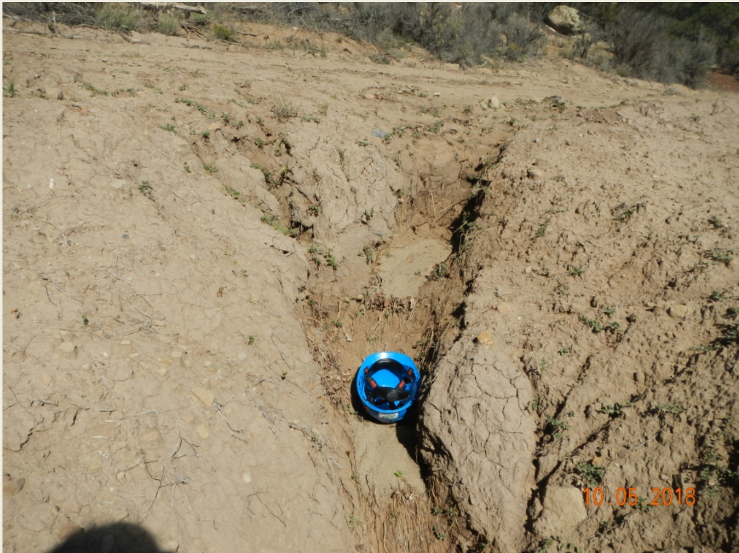
Photo 9. View of erosional channel up to approximately 2.5 feet wide and 1.5 feet deep from stormwater flows off of the access road.
