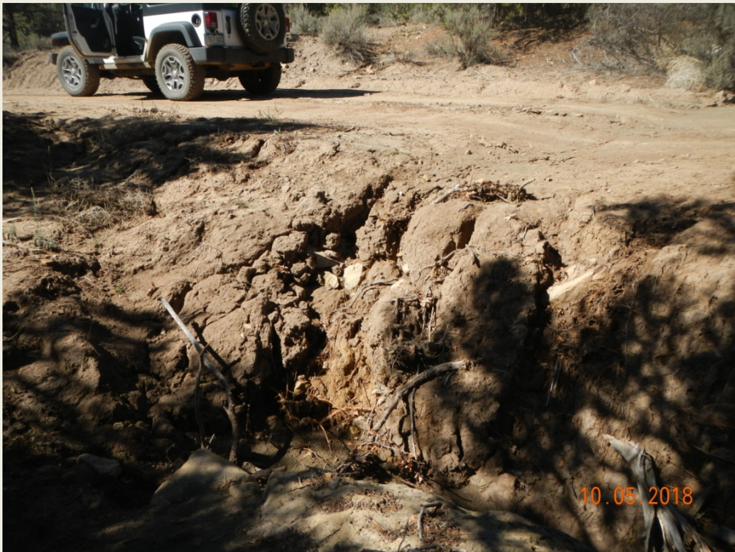
Photo 10. View of the another erosional channel where stormwater flows over the access road resulting in deep rilling and erosional channeling down-slope from the access road.
