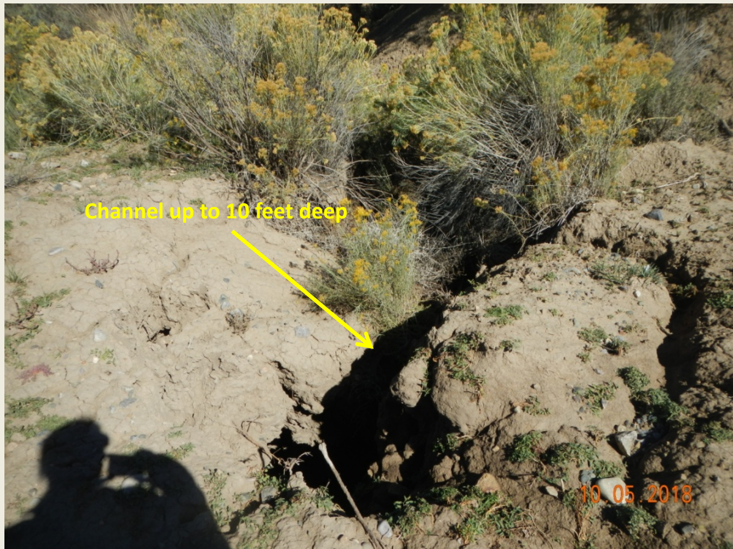
Photo 12. View of area downslope of Photo 12, where stormwater flows from the access road surface are eroding the bank of La Boca Creek, erosional channels up to 10 feet deep and 4 feet wide. Area where access road crosses over creek needs stabilization.
