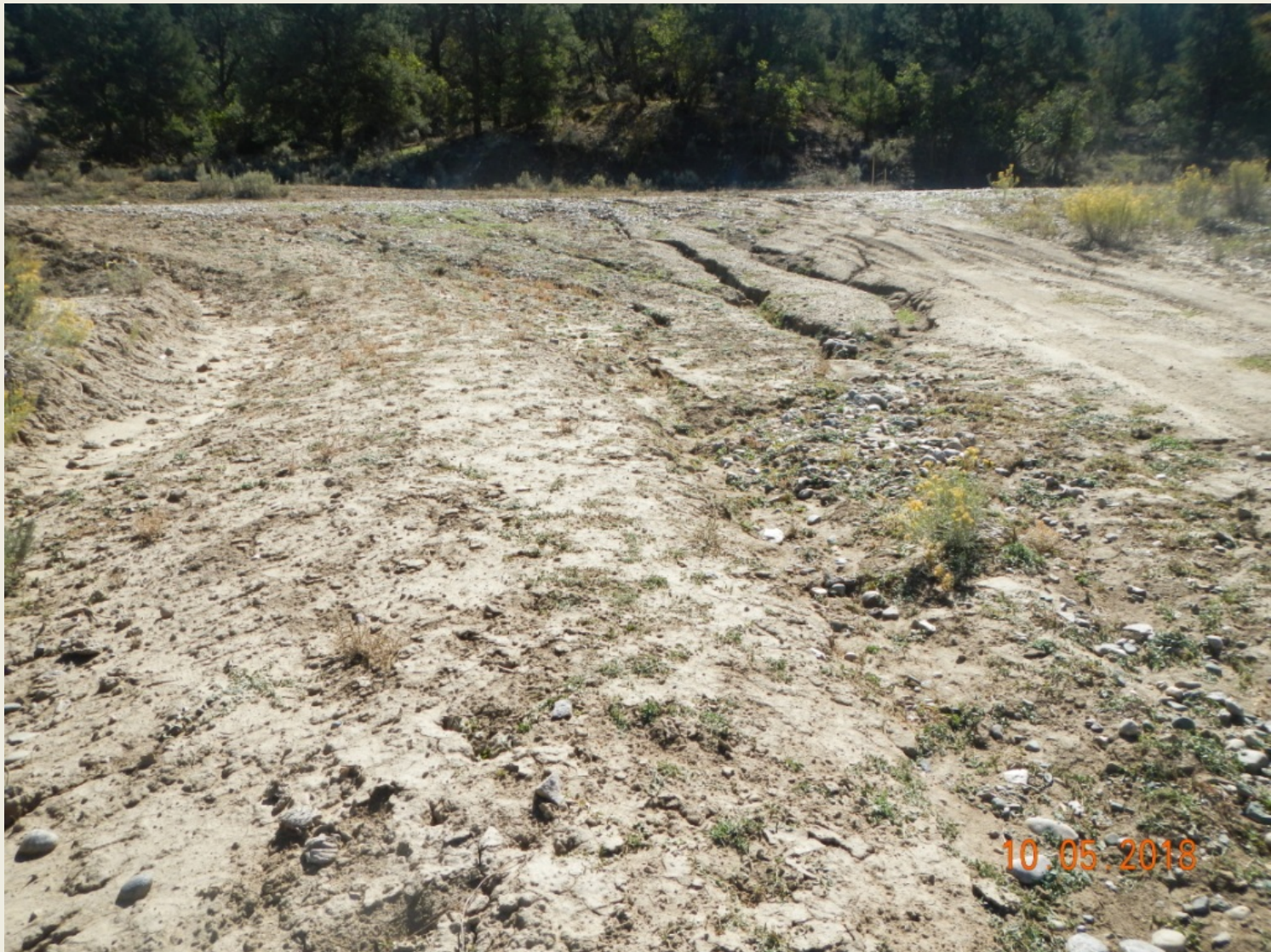
Photo 11. View of area at the beginning of the access road where stormwater is eroding a channel into the road base toward La Boca Creek.
