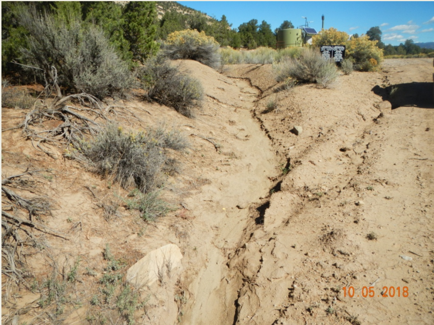
Photo 7. View of erosional channeling near the well pad entrance, north of access, where diverted stormwater from the well pad is not properly de-energized, and soils are not stabilized, resulting in erosional channeling and sediment deposition and transport off of the project area.
