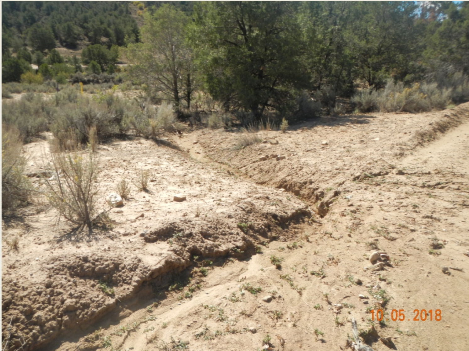
Photo 8. Downstream view of erosional channel, diverted from the well pad that is not properly stabilized or de-energized resulting in erosion and sediment deposition/transport south from the project area.
