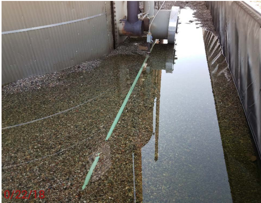
Location Photo #5, battery containment has seasonal water in it.
