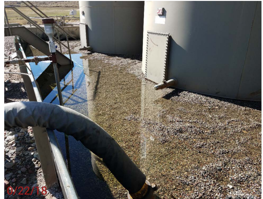
Location Photo #6, battery containment has seasonal water in it.
