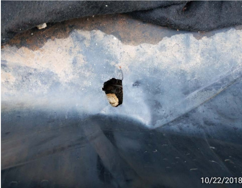
Hole in bottom of berm liner
