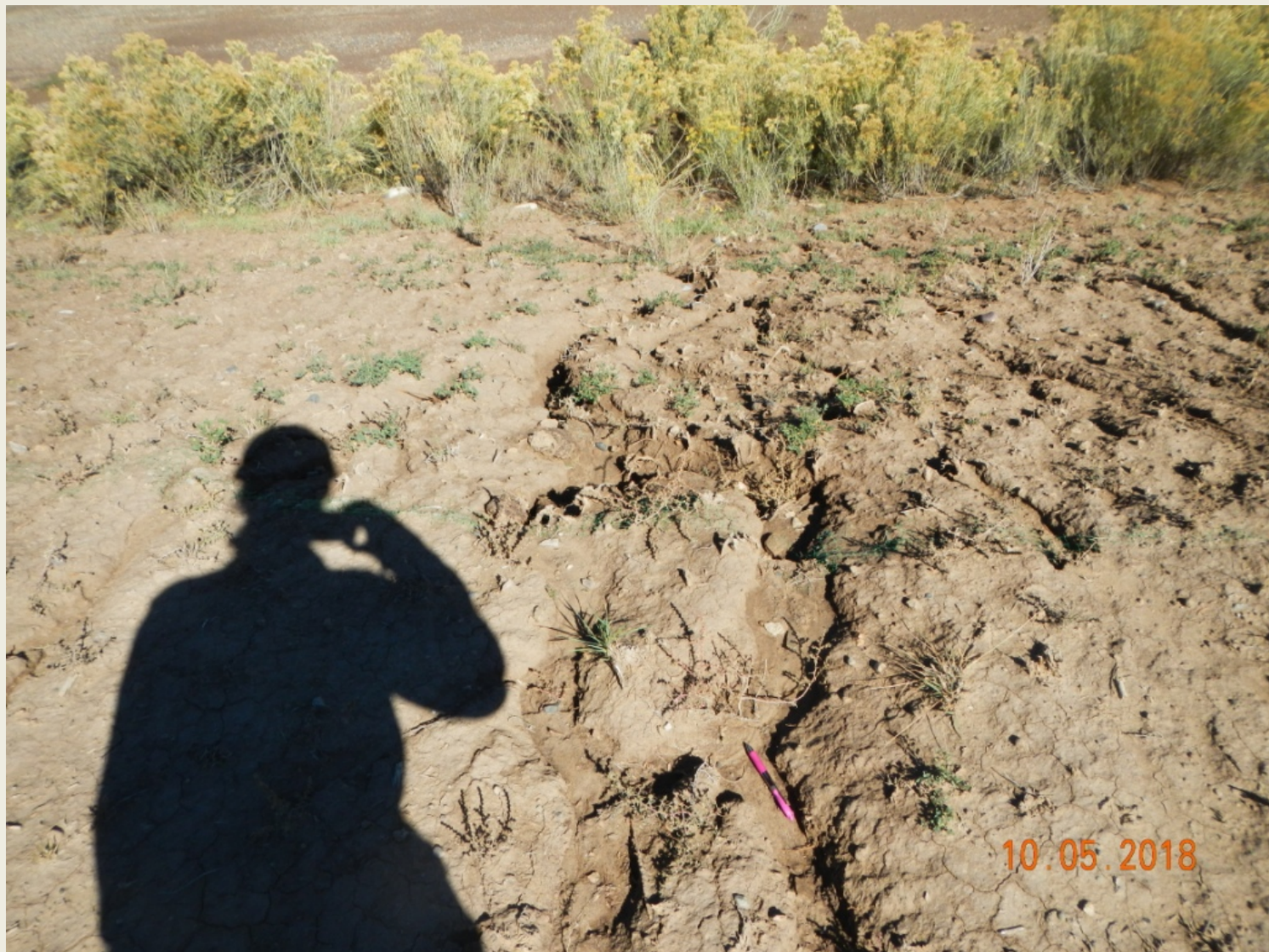
Photo 7. View of more rilling up to 12 inches deep in the central fill slope.
