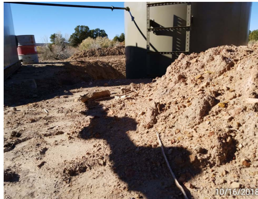
No berm around ¼ of tank
