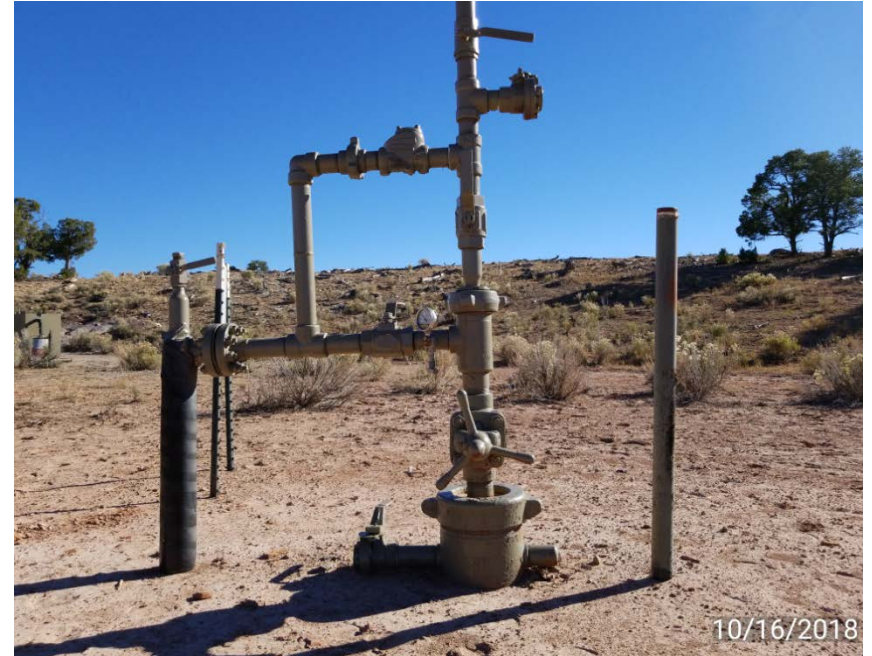
Riser next to well head not plugged or locked out tagged out
