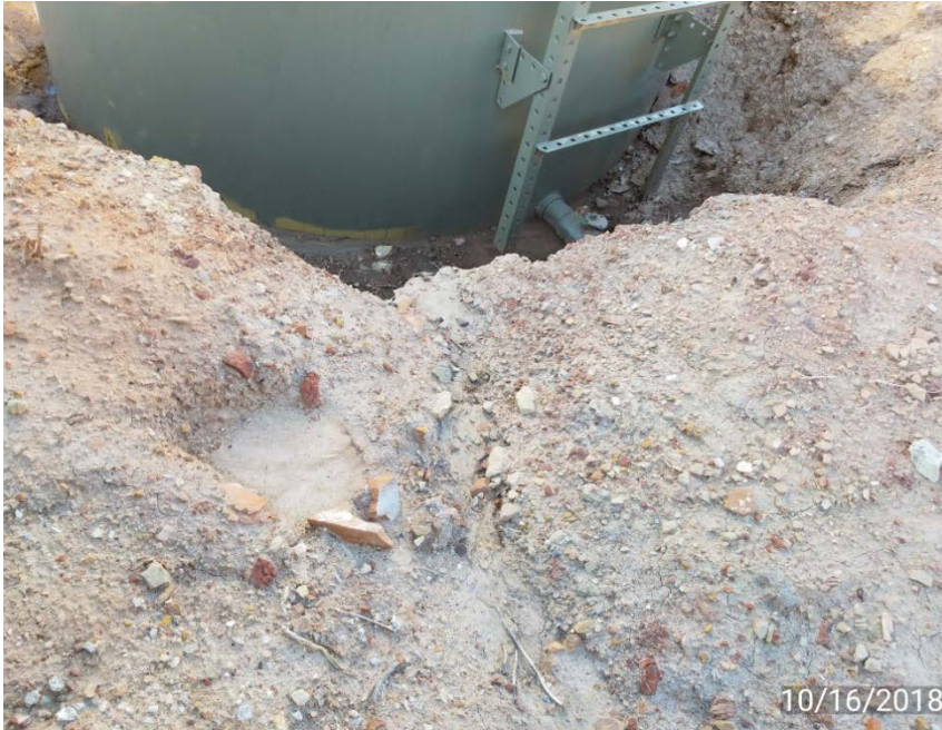
Storm water entering around tank where berm doesn't exist
