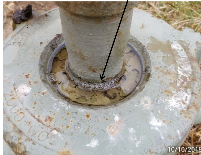
Gas leakage at well head around tubing
