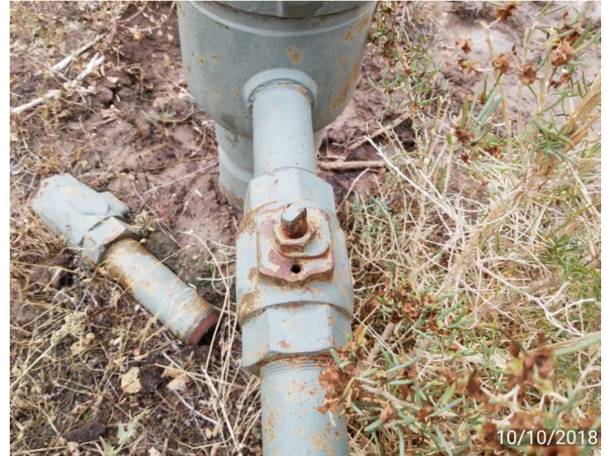
Casing valve partially open
