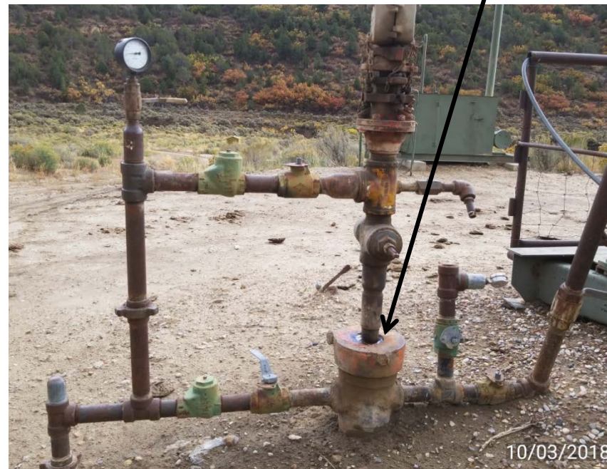
Gas leaking at well head
