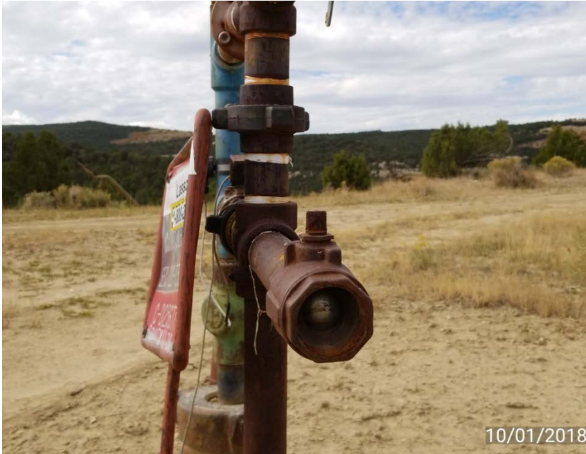
Pipe at well head without cap.
