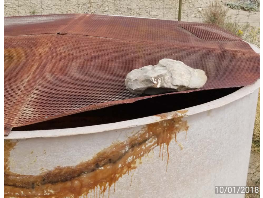
Hole in cover of pit tank
