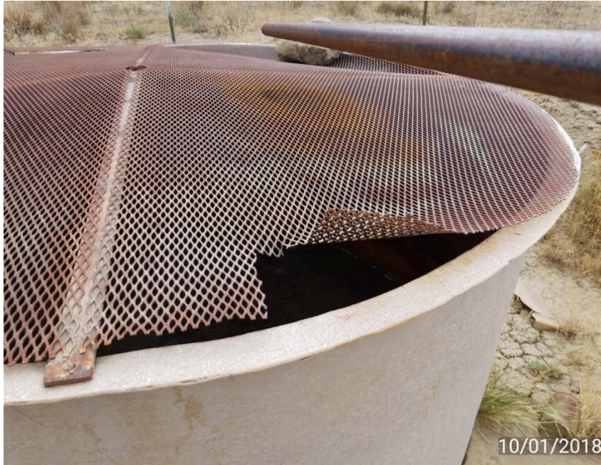
Hole in cover of pit tank
