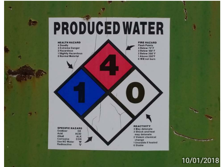
Tank sign missing 100 bbl tank capacity, operator, and emergency contact number.
