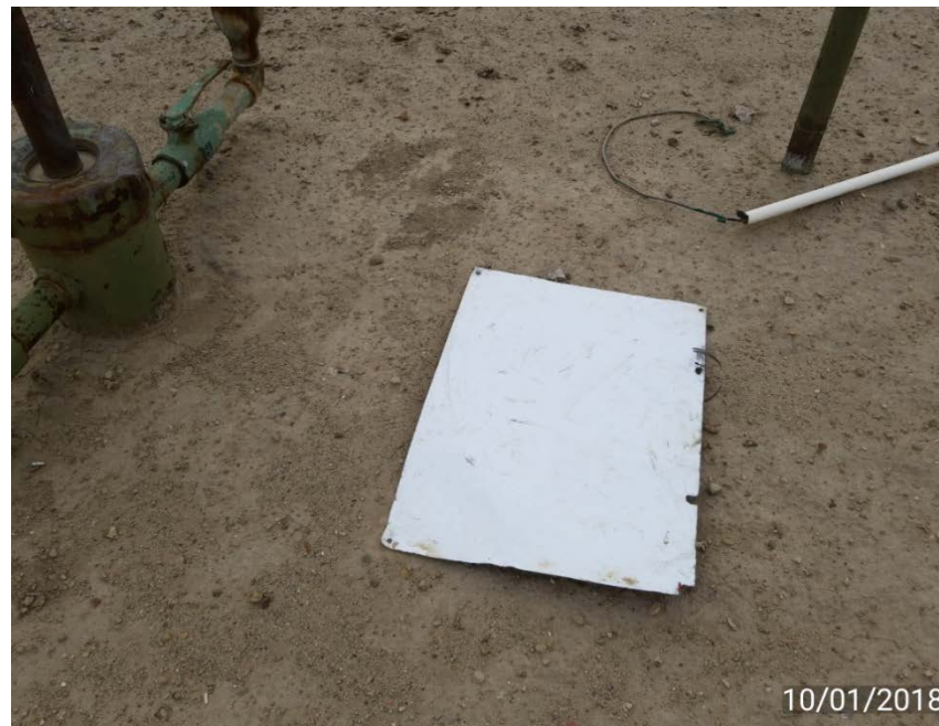
Well sign detached from wellhead.
