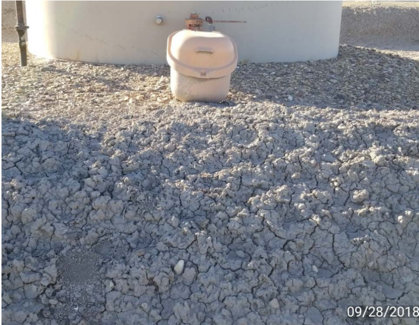
Berm worn down by off loading valve
