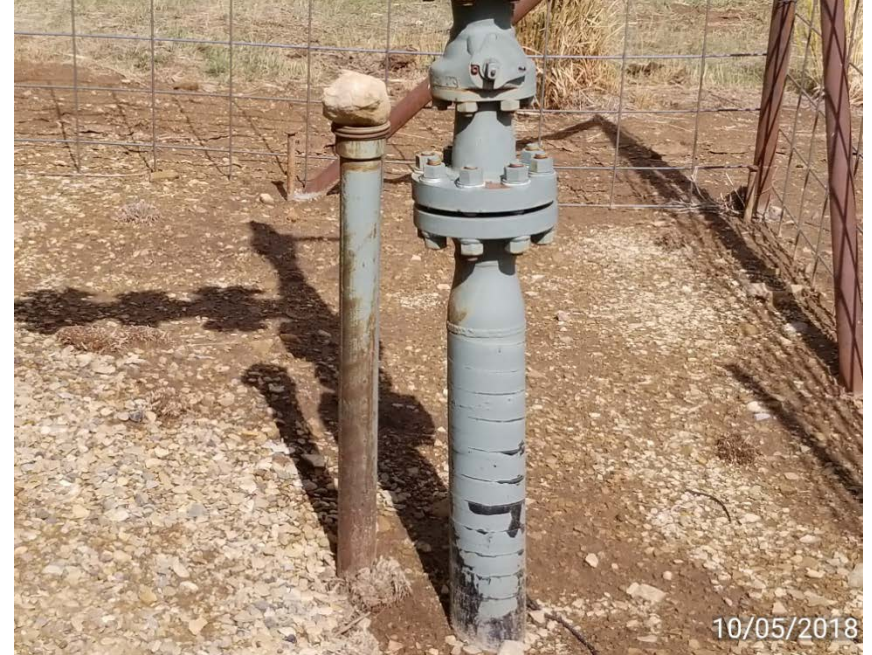
Riser without end sealed or locked out tag out. Located next to building.
