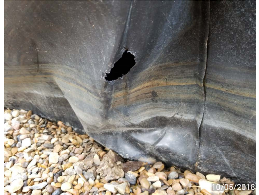
Hole in tank battery liner
