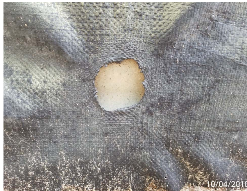
Hole in berm liner
