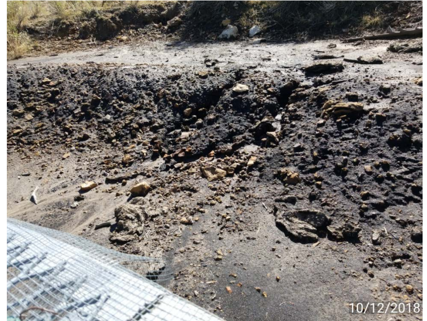
Storm water has washed out berm on uphill side.
