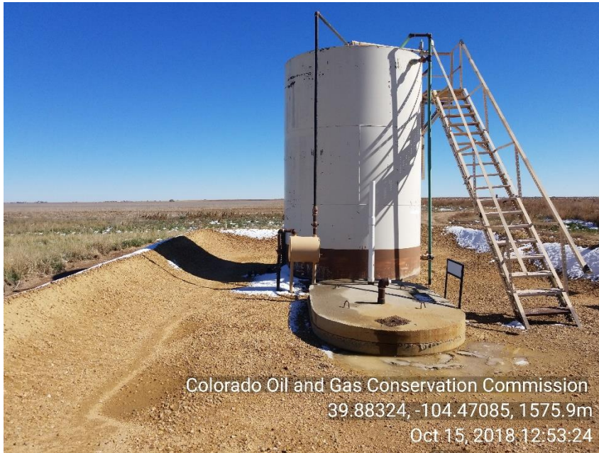
Photo 3 Knock out tank to ECD off crude oil tank
