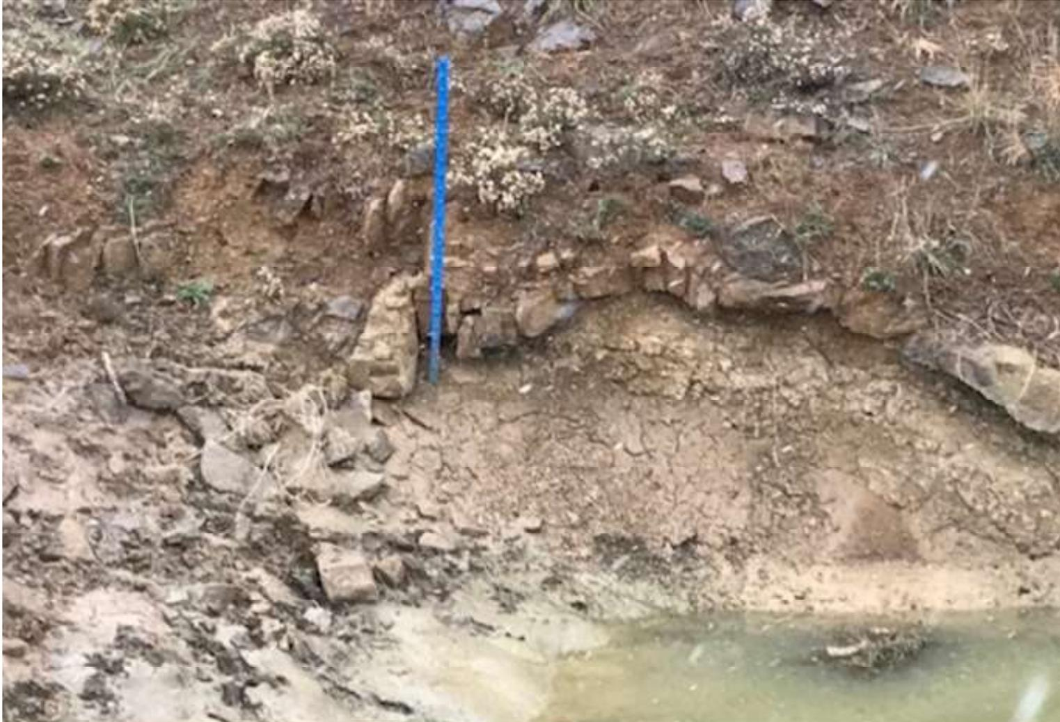
THE PRODUCED WATER WAS PULLED FROM THE PRODUCTION PIT TO PROVIDE (2) FEET OF FREEBOARD, IN COMPLIANCE WITH RULE 902.b.
