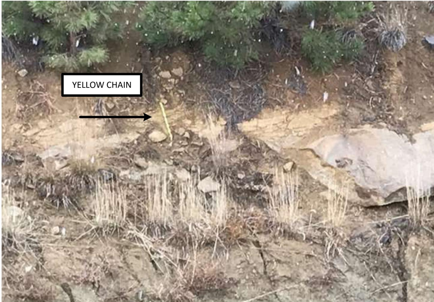
A YELLOW CHAIN WAS INSTALLED IN THE PRODUCTION PIT TO MONITOR (2) FOOT OF FREEBOARD BETWEEN THE TOP OF THE PIT WALL AND THE FLUID LEVEL OF THE PIT.
