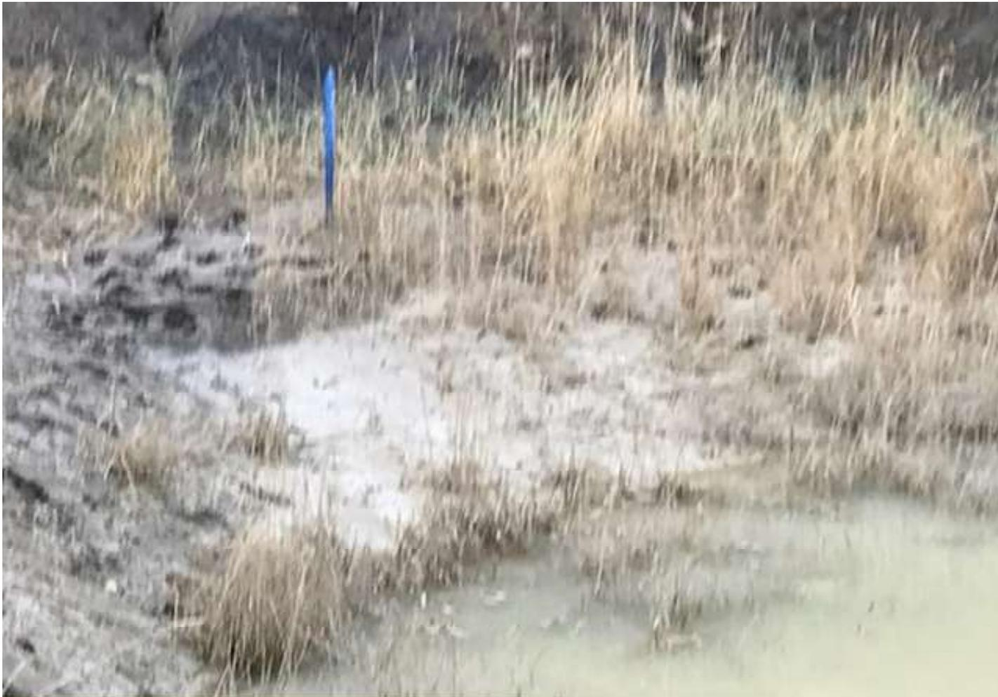
THE PRODUCED WATER WAS PULLED FROM THE PRODUCTION PIT TO PROVIDE (2) FEET OF FREEBOARD, IN COMPLIANCE WITH RULE 902.b.
