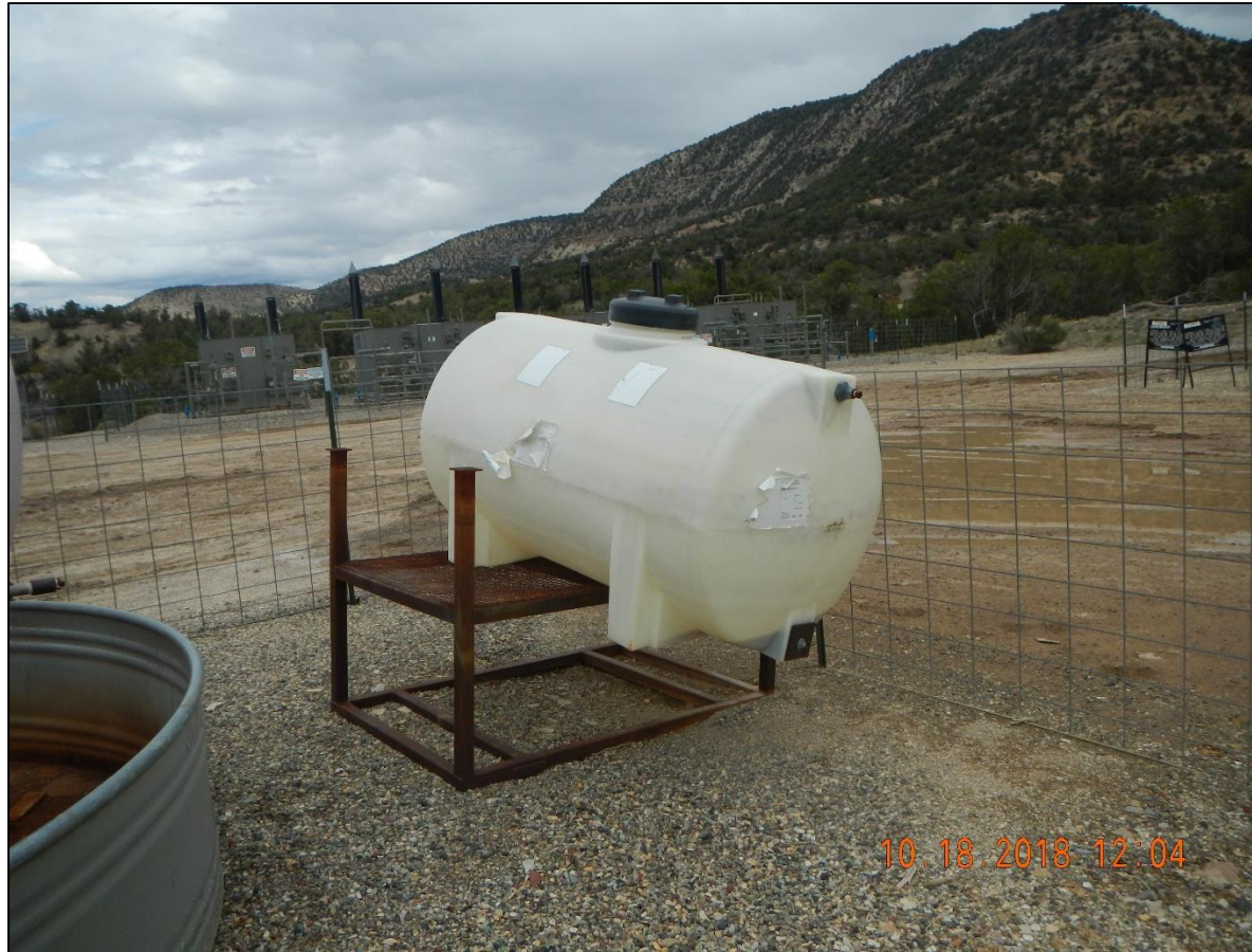
Unused container with no readable label and no secondary containment.
