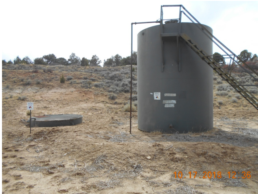
Tank battery. Berms need maintained
