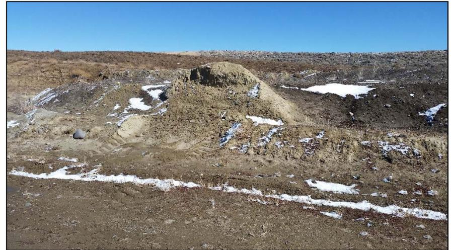
**Photo 2. Cuttings berm pushed in; compromised.**
