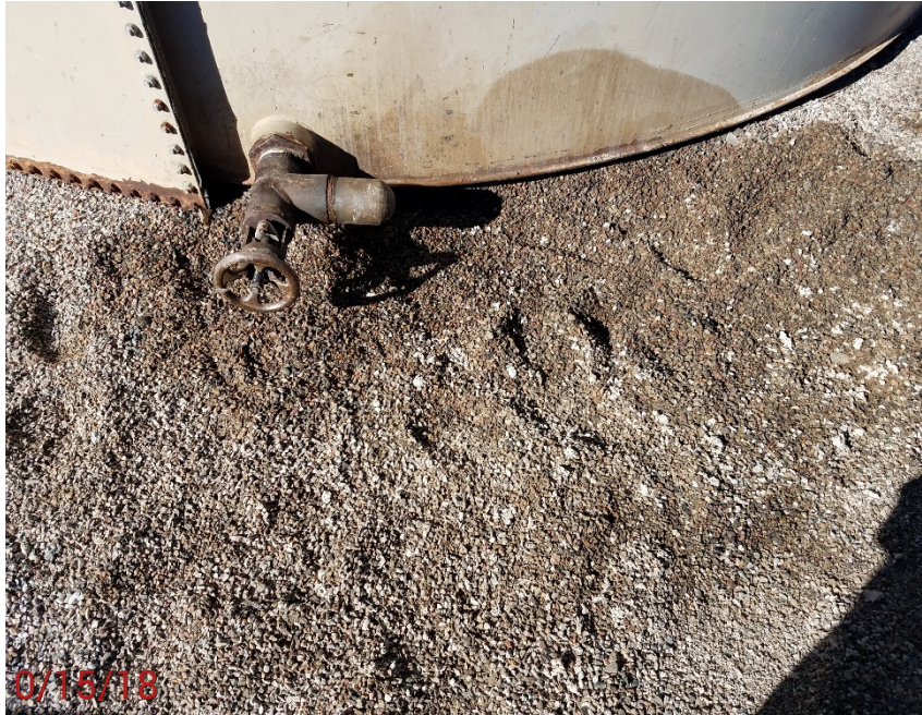
Location Photo #5, Oily stained rock in battery containment.
