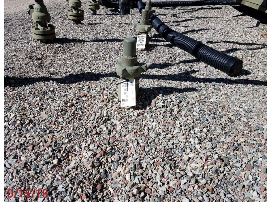
Location Photo #6, 4 unused flow line risers
