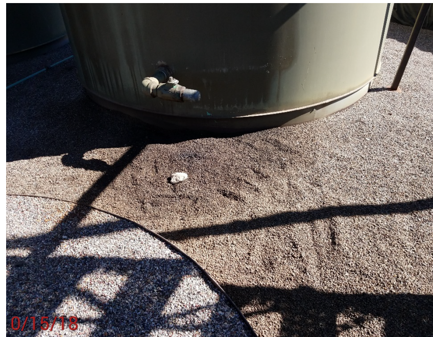
Location Photo #10, Stained rock in battery containment.
