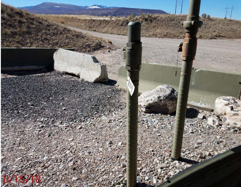
Location Photo #5, unused flow line riser
