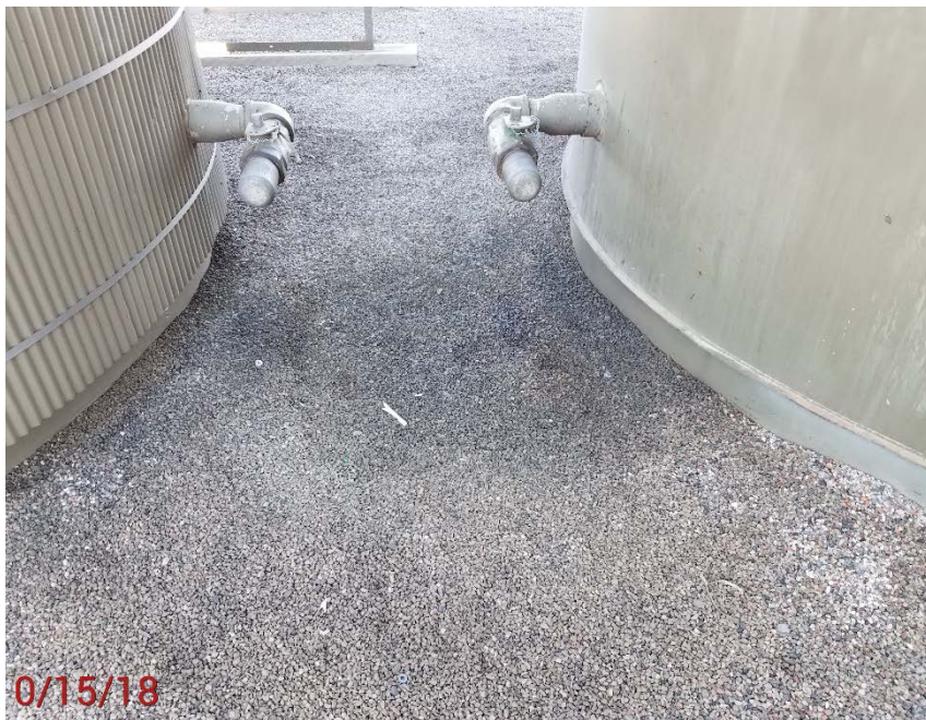
Location Photo #11, Stained rock in battery containment.
