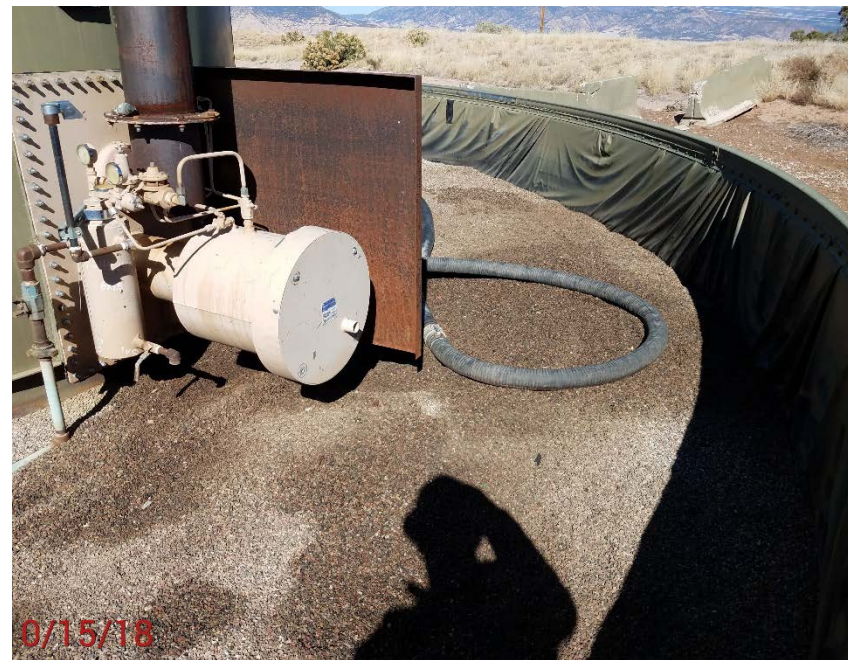
Location Photo #12, , Stained rock in battery containment.
