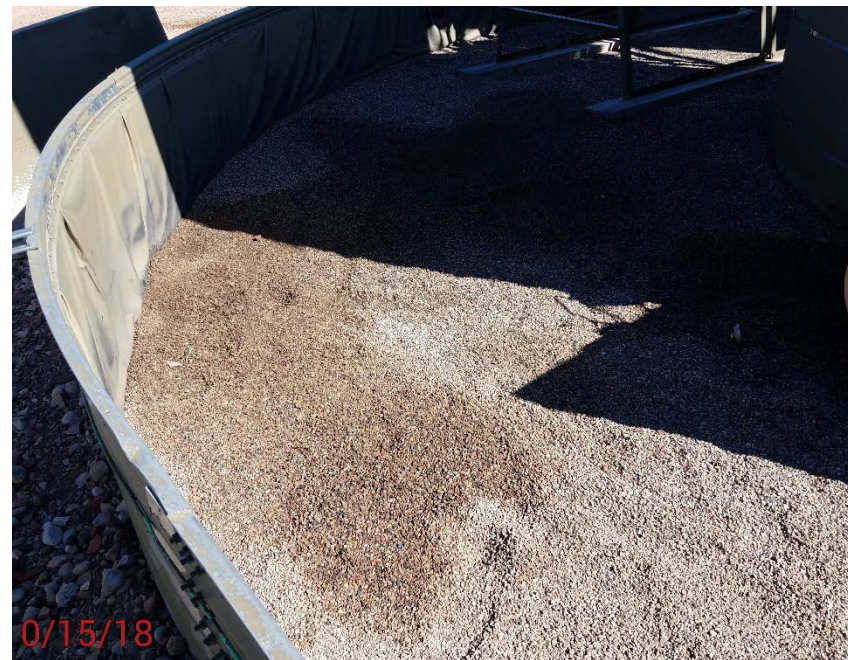
Location Photo #8, Stained rock in battery containment.
