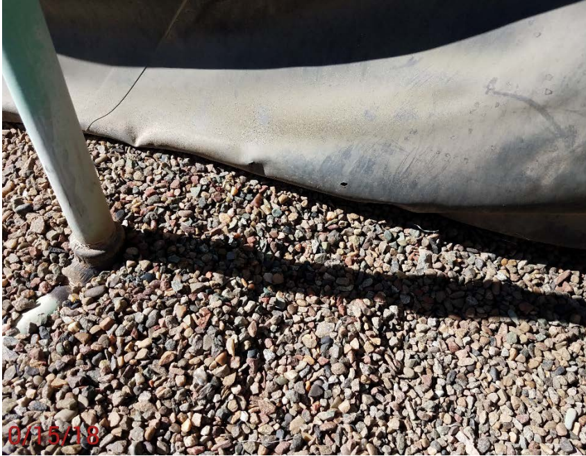
Location Photo #3, holes in secondary containment
