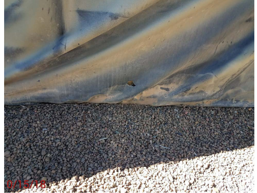
Location Photo #4, holes in secondary containment
