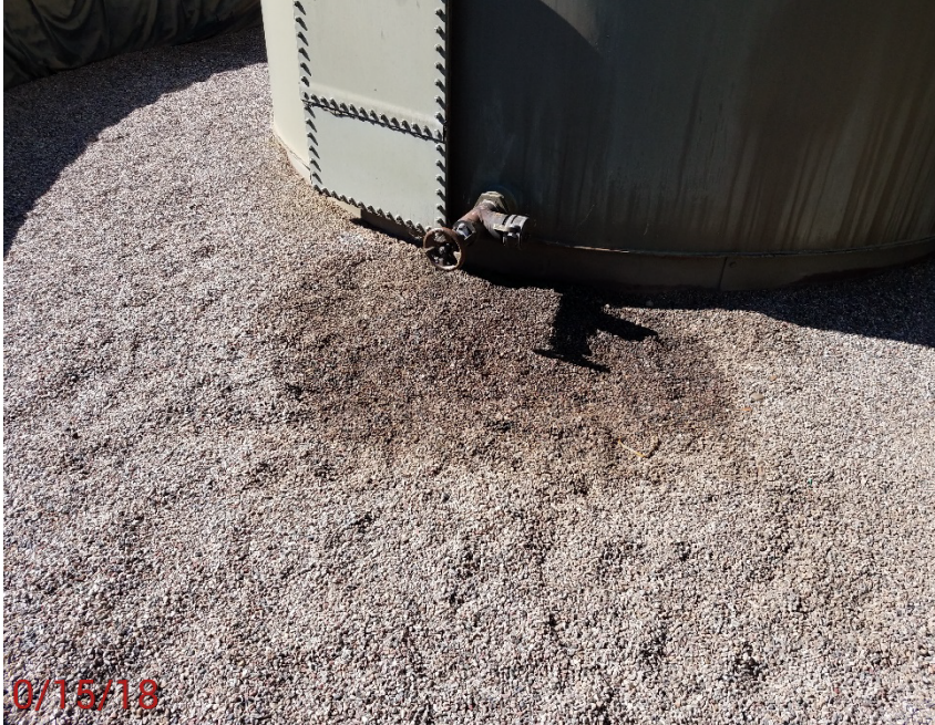
Location Photo #13, Stained rock in battery containment.
