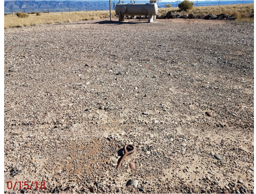
Location Photo #6, Unmarked deadman East end of location.
