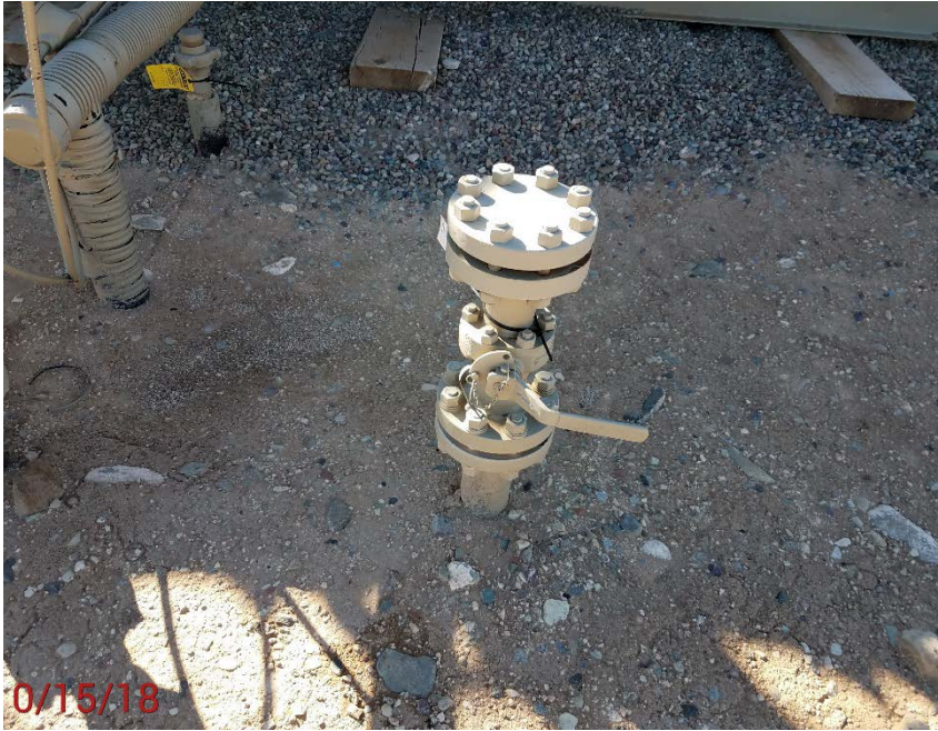
Location Photo #5, unused flow line riser
