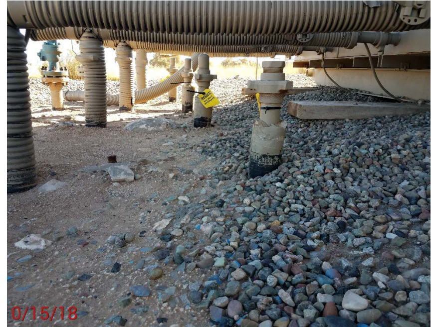
Location Photo #4, Unused flow line risers
