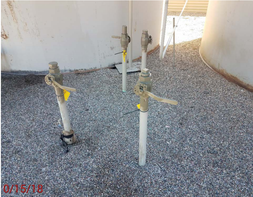
Location Photo #3, Unused flow line risers
