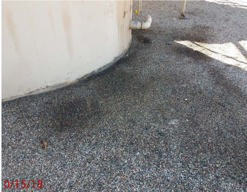
Location Photo #7, Stained rock in battery containment.
