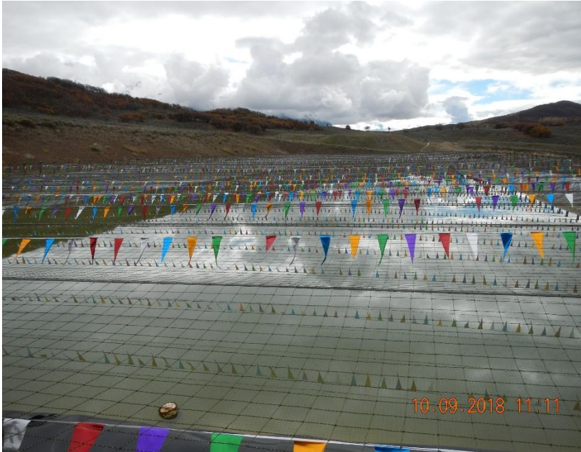
Upper Pit (#4), Facility ID #418790. Fence and netting are in good condition.
