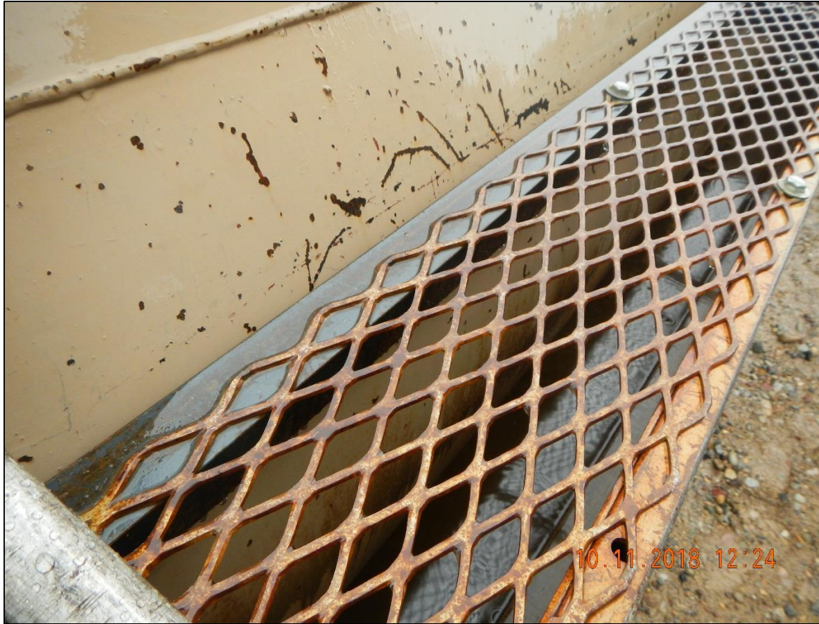
Fluid in secondary containment
