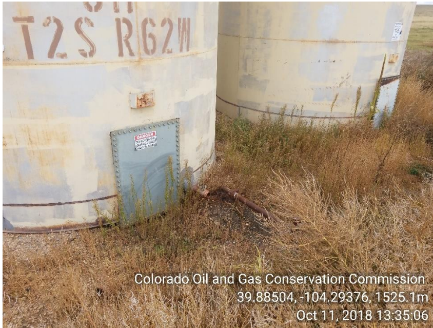
Photo 7 Leaking 2" inlet pipe to crude oil tank not connected
