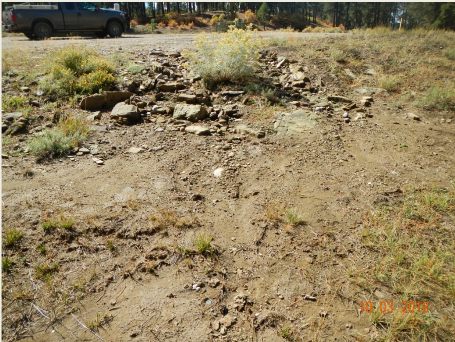
Photo 3. View of area in the northwestern project area where stormwater flows off of the well pad, scouring the rocky upper portions, and depositing sediment down-slope.
