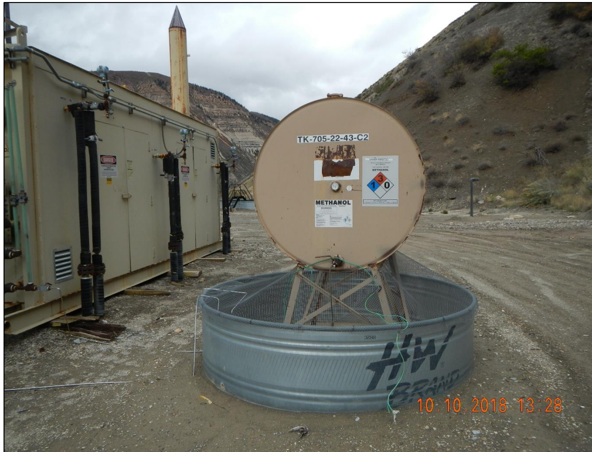
Methanol tank with rusted out secondary containment base.
