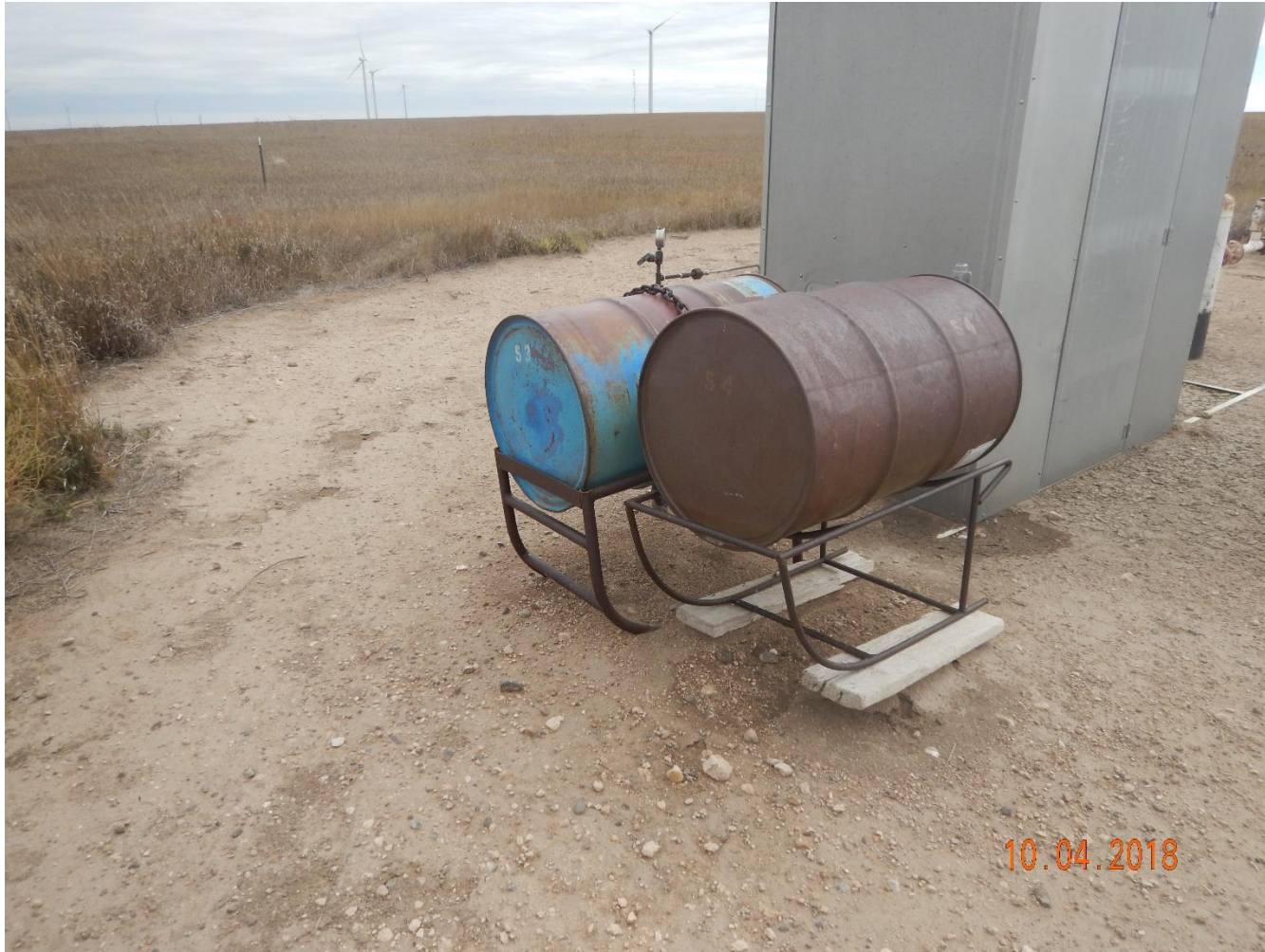
Photo 3: Photo taken from the meter shed, southwest of the well (40.905553/-103.247635). Photo shows two barrels without secondary containment.
