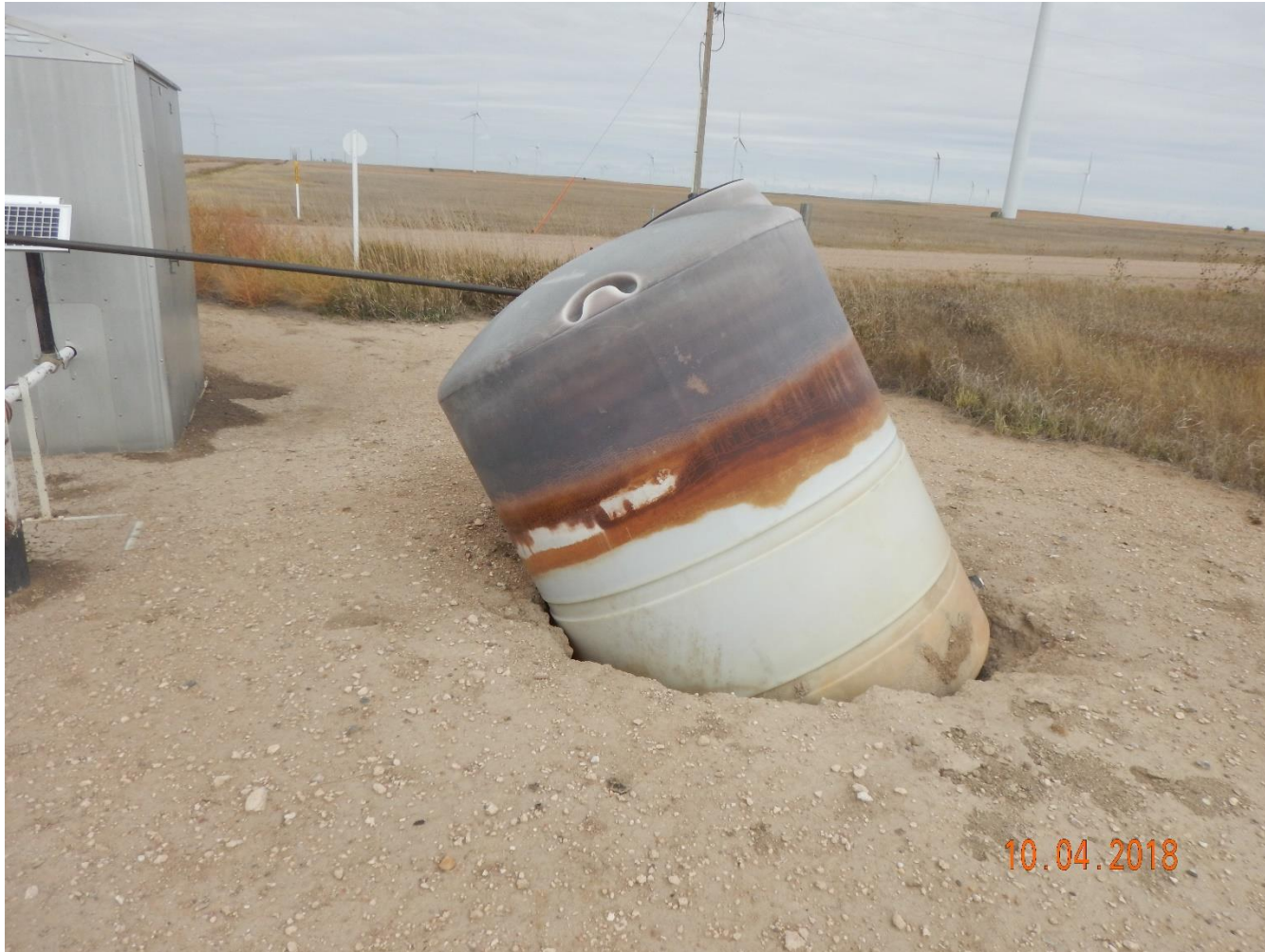
Photo 4: Photo taken from the meter shed, SE of the well. Photo shows fiberglass tank that appears to have tipped over.
