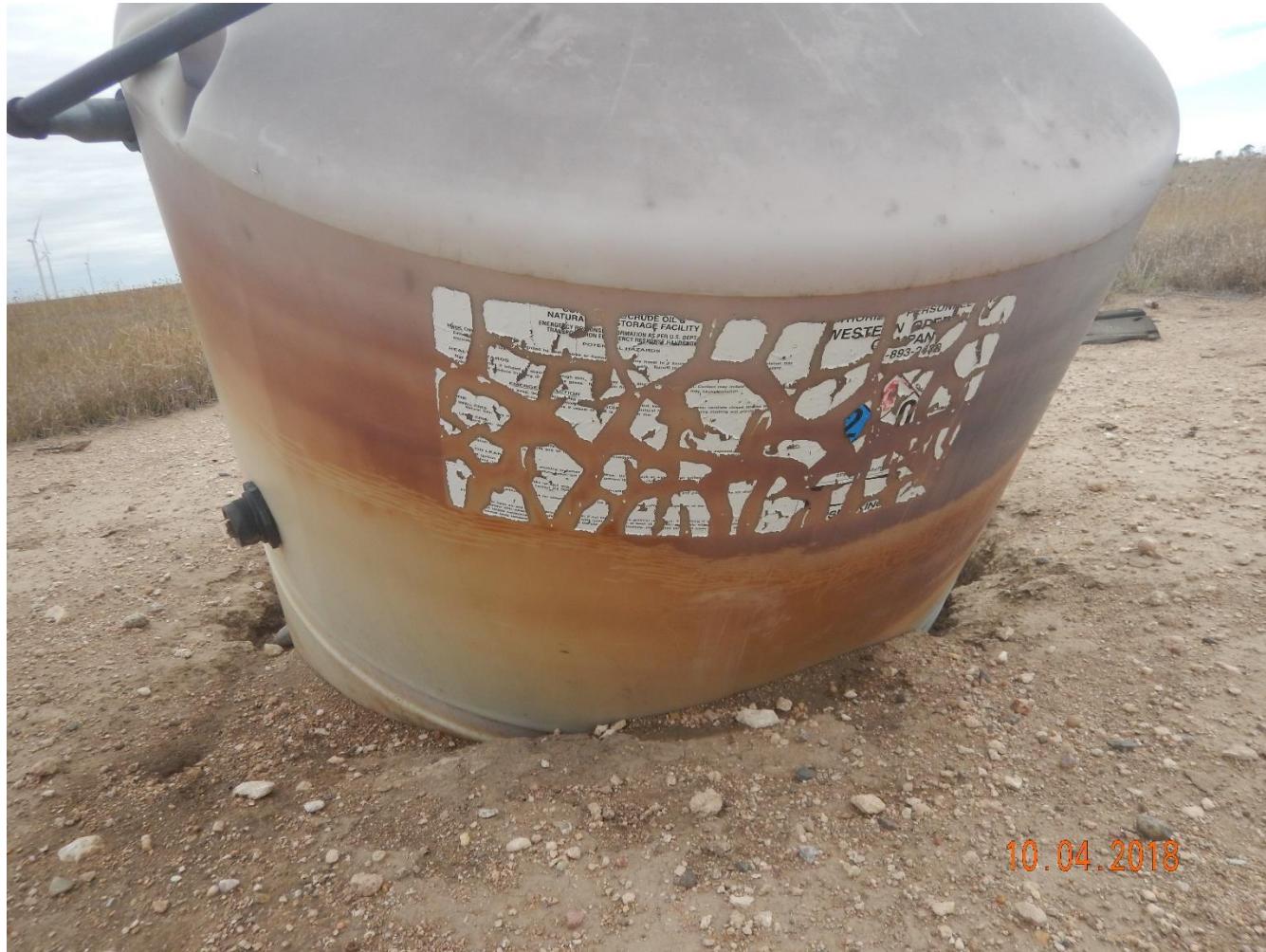
Photo 5: Continued from photo 4. Photo shows tank without appropriate labeling.
