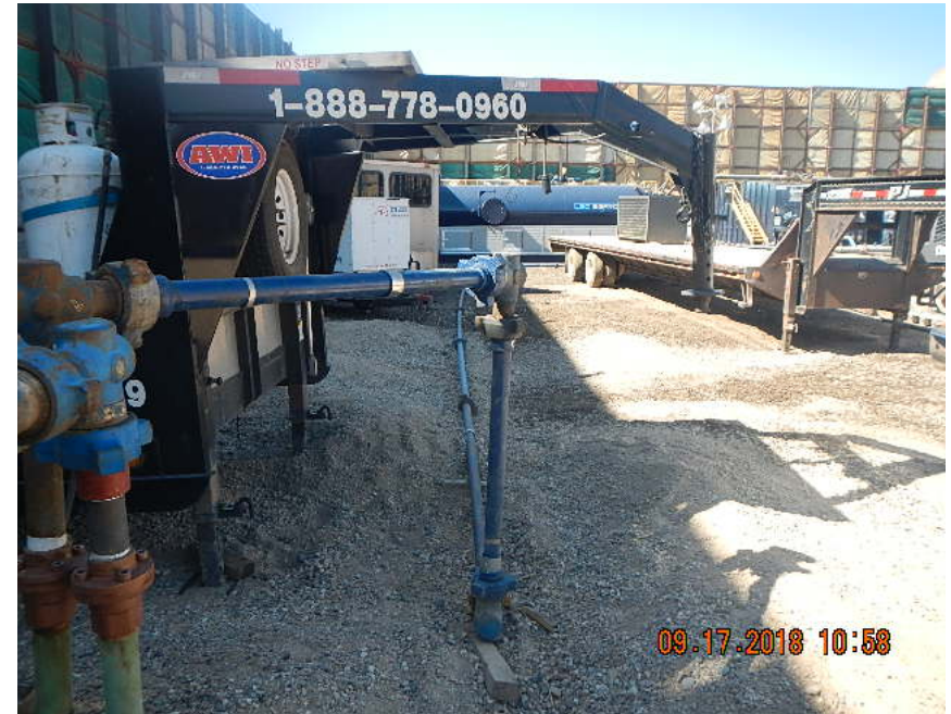
Flow line riser to P Tank separator unit.
