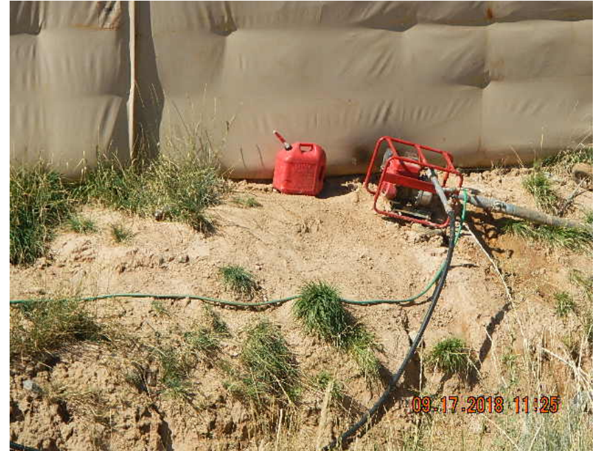
Fuel tank outside of sound walls, No containment or labels.
