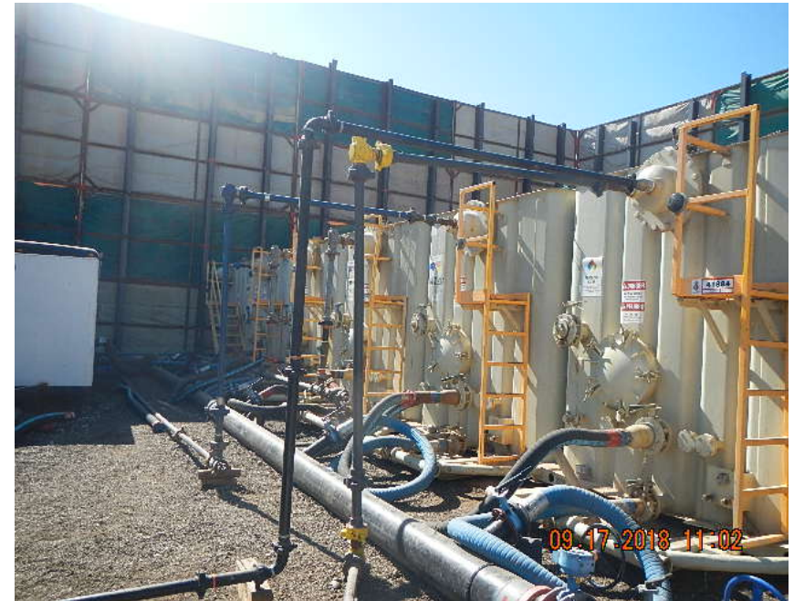
Flow line from P Tank to flow back tanks
