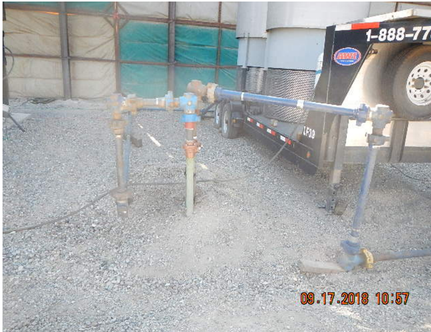
2 risers from separator units, no production tanks on this location
