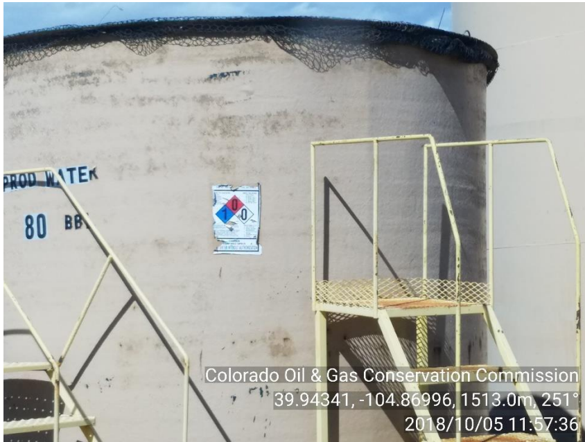
PHOTO 7: NFPA PLACARD ON PRODUCED WATER TANK
