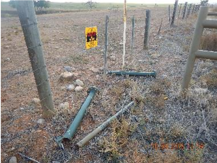
Photo 5: Disconnected vent stacks on SE fence line.
