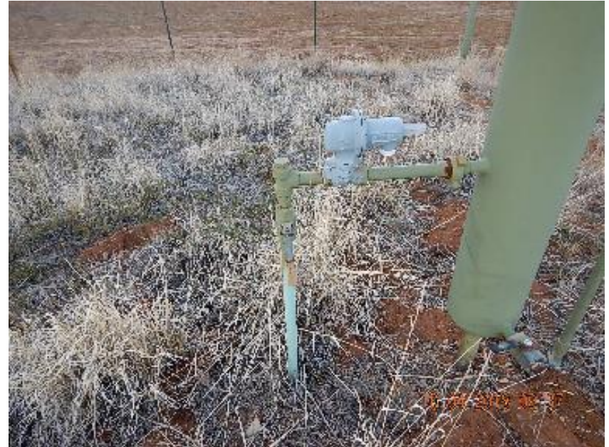
Photo 4: 1" steel supply gas line to domestic tap. Unable to locate (A) point.
