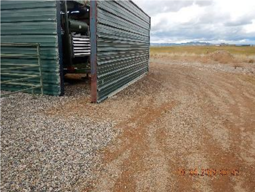
Photo 3: Angle iron along base of sound wall.
