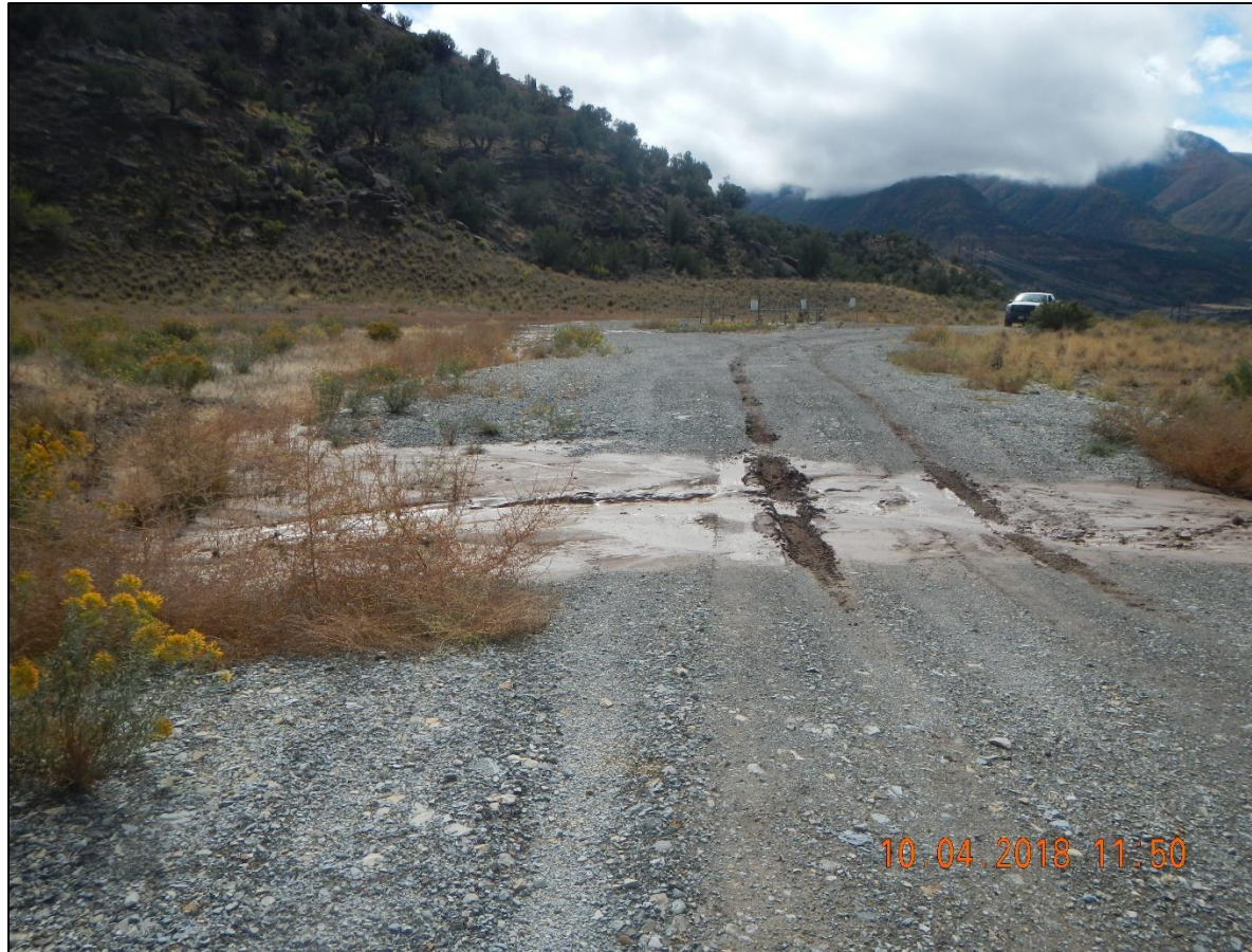
Sediment build up in low water cross.
