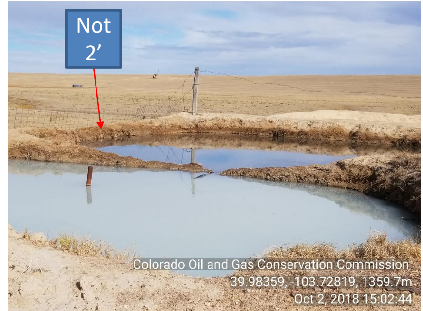
Photo 8 Loc pit does not have 2' of free board
