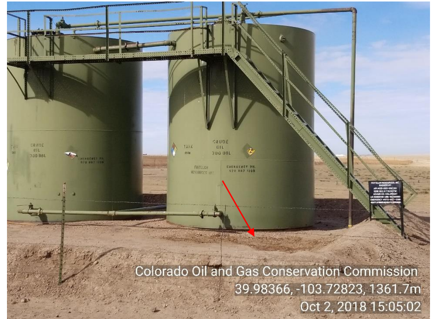
Photo 4 TNK BTRY stained soil in front of crude oil tank.
