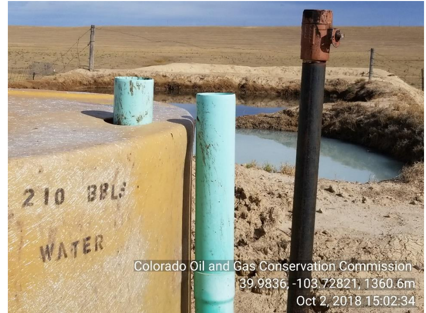
Photo 6 Produced water tank no placard
