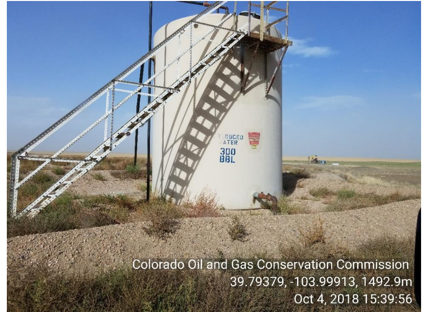
Photo 4 Produced water tank no placards
