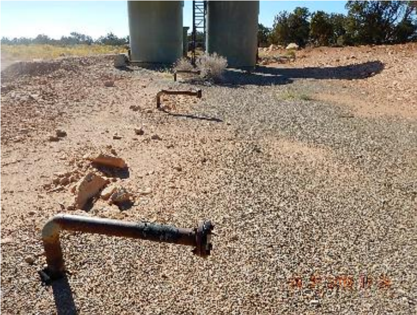
Photo 9: Risers inside tank battery containment.
