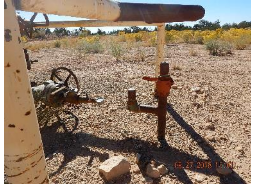
Photo 2: Steel riser at wellhead.
