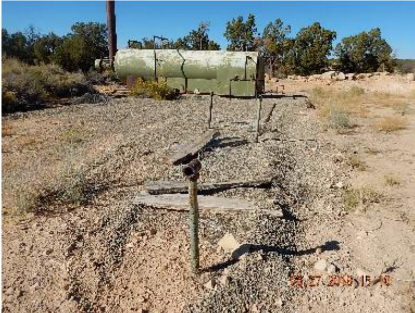
Photo 3: Steel risers at heater treater.
