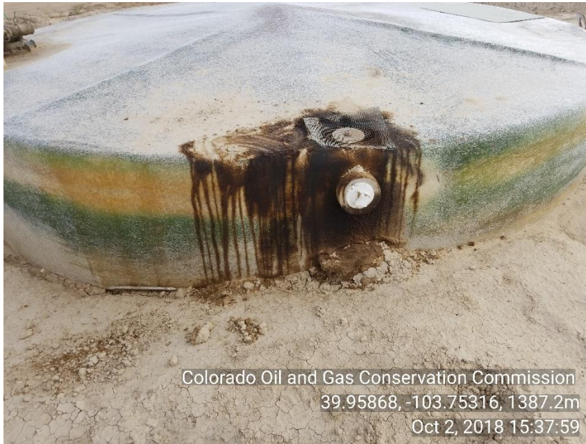
Photo 9 stained soil improper tank lid
