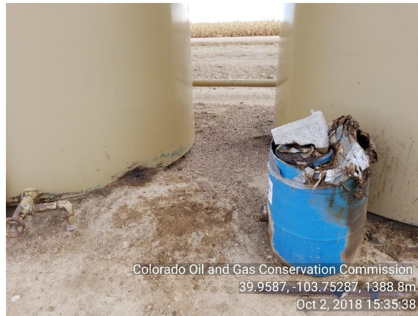
Photo 6 Stained soil and trash around crude oil tank
