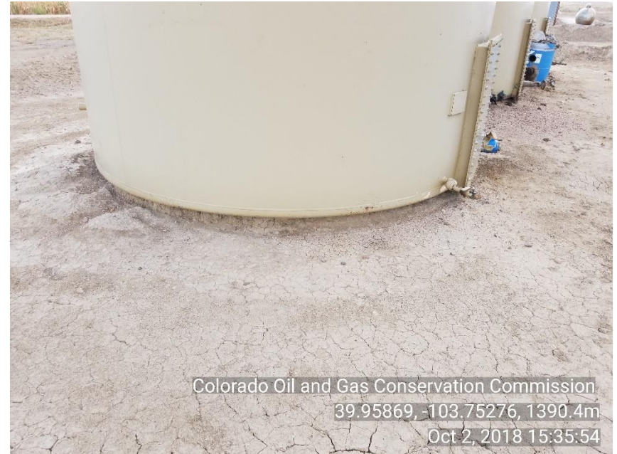
Photo 4 Erosion under 300BBL oil tank
