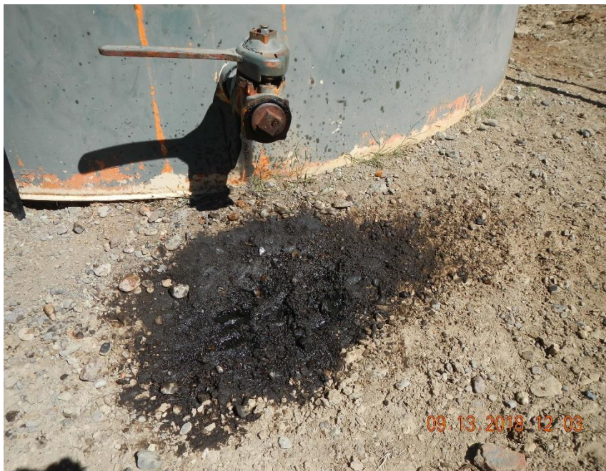
Stained soil beneath truck load out valve on AST.
