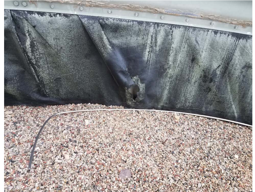
Location Photo #8, Holes in secondary containment.
