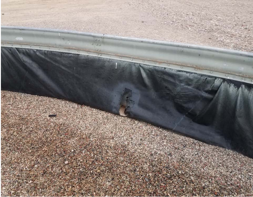
Location Photo #9, Holes in secondary containment.
