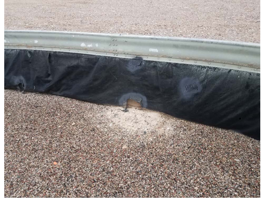
Location Photo #12, Holes in secondary containment.
