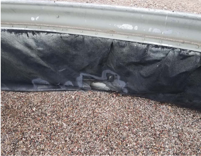
Location Photo #11, Holes in secondary containment.
