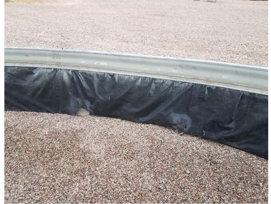
Location Photo #10, Holes in secondary containment.
