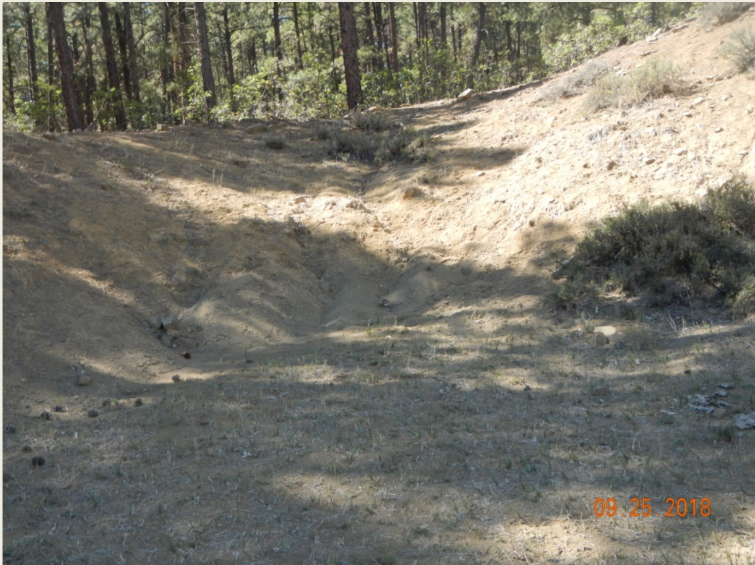
Photo 6. View of the southwestern corner of the project area where stormwater run-on is eroding the well pad cut-slope and depositing sediment down-slope.
