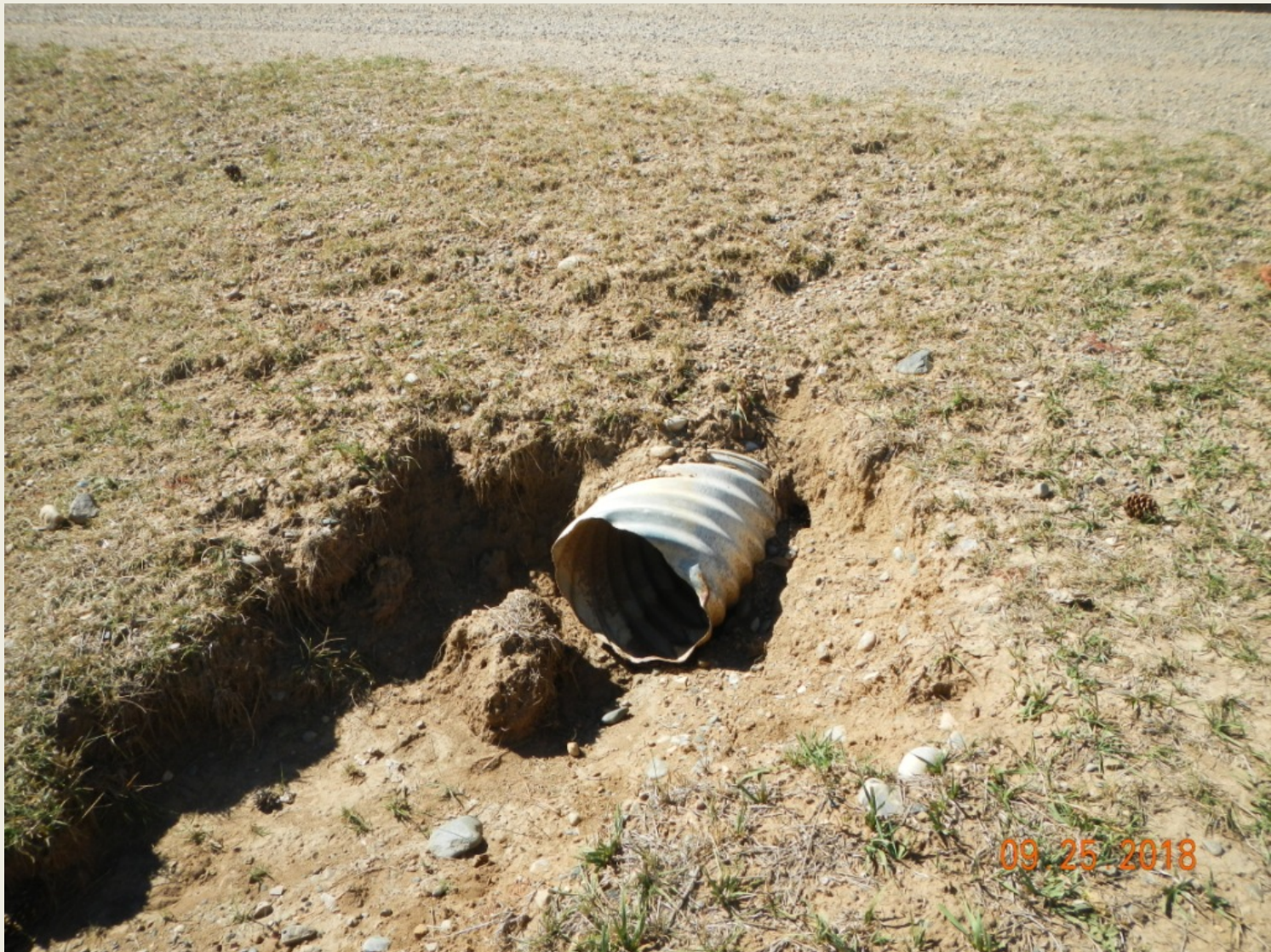
Photo 5. View of erosion at culvert outlet in southeastern project area.
