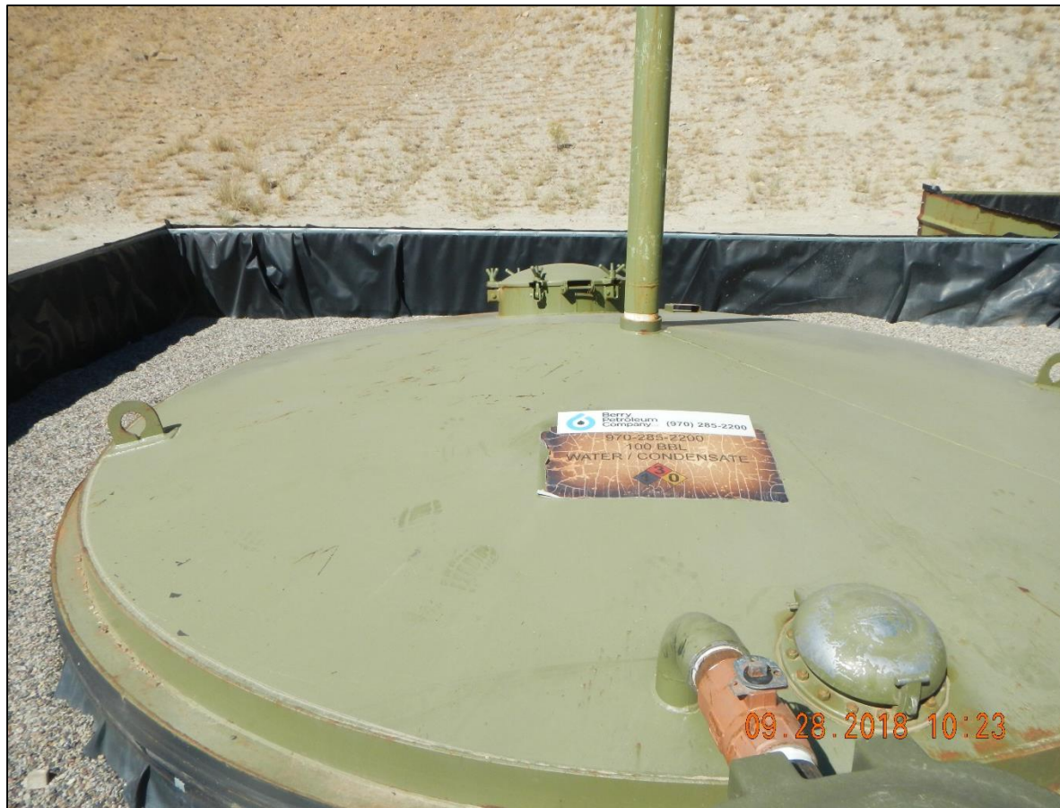
Peeling, cracking, and discoloring of tank label.
