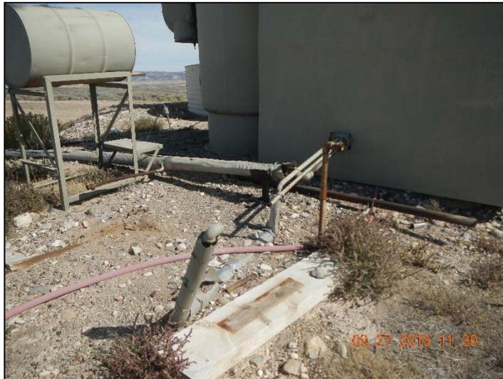
**Photo 3. 2 unmarked risers adjacent to separator.**
