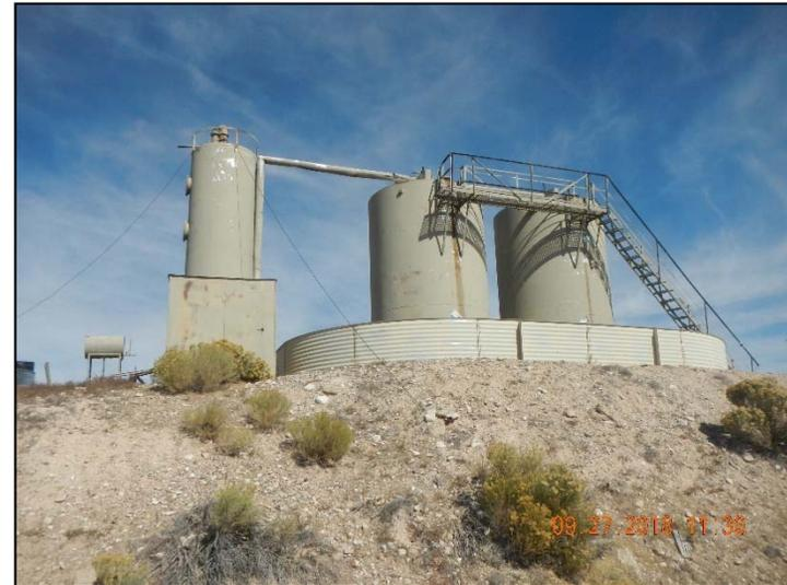
**Photo 4. Separator less than 50 feet from fired tanks.**
