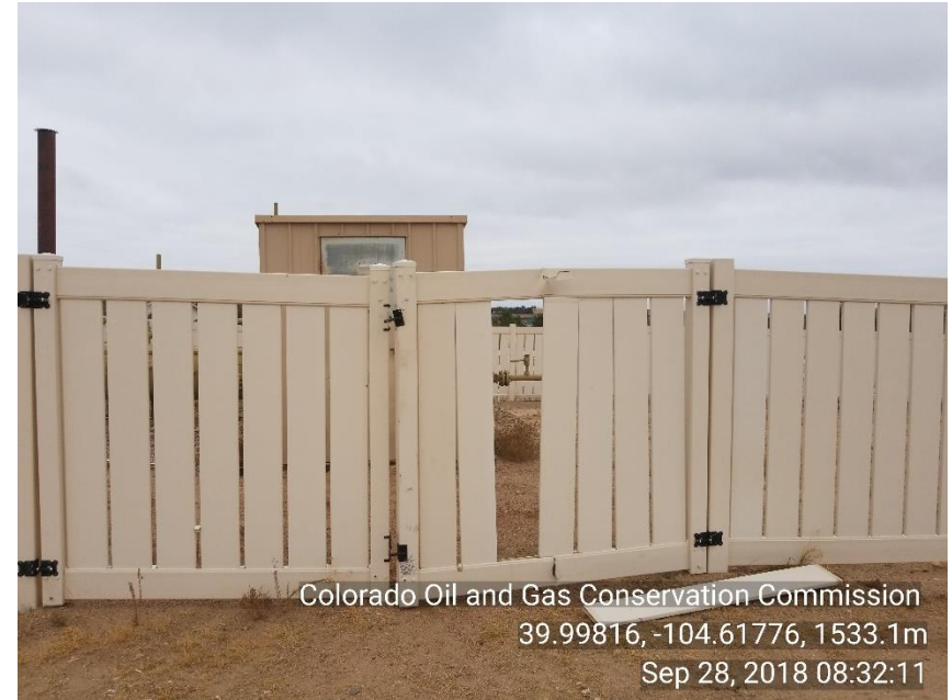
Photo 6 Broken gate with missing Panel
