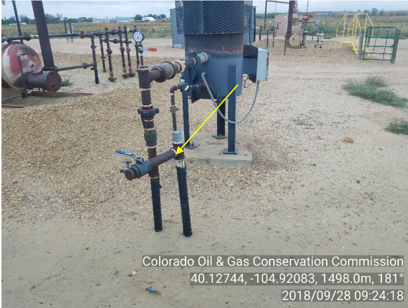
PHOTO 5: UNMARKED RISER
