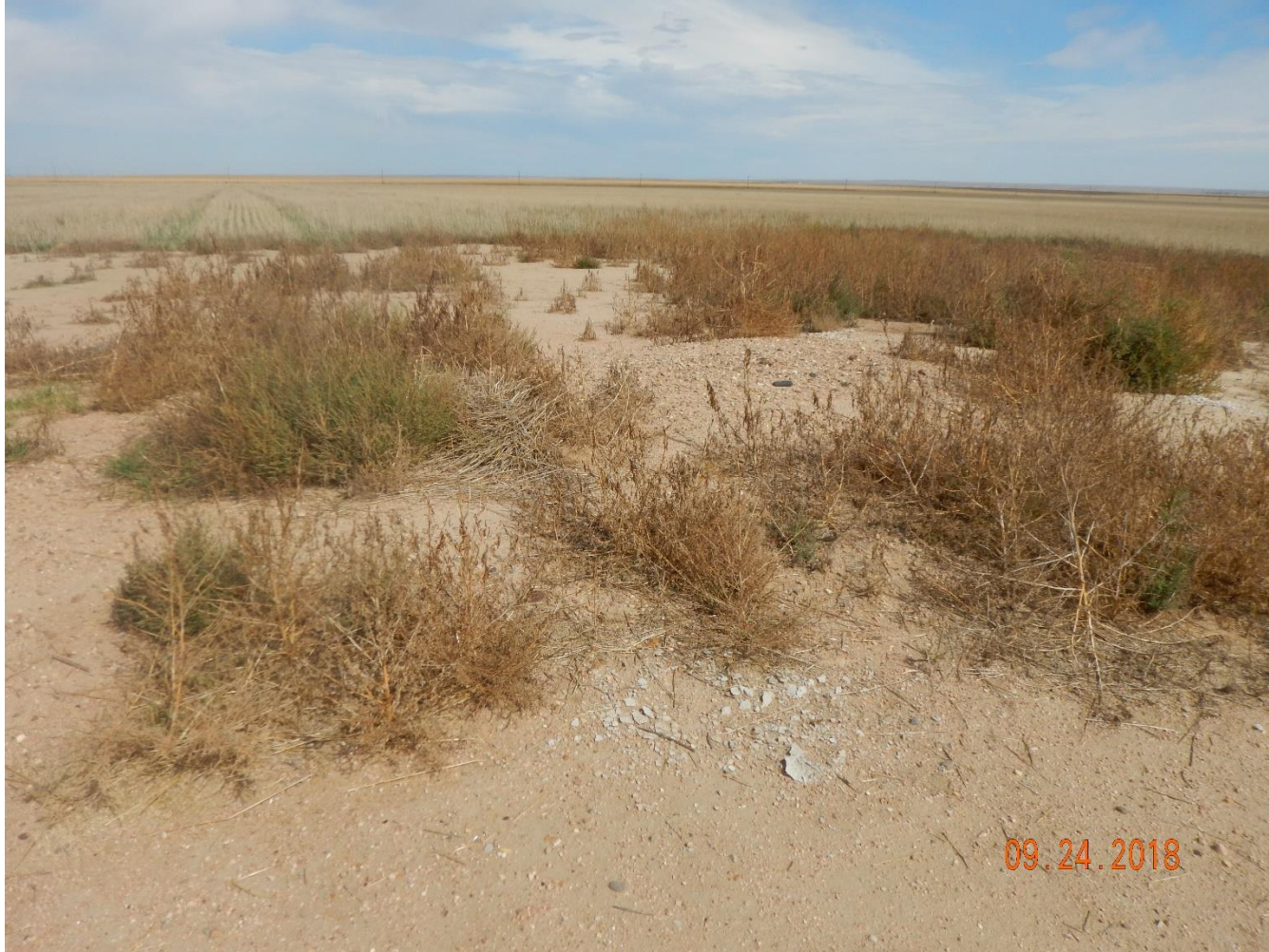
Photo 4: Photo taken the well location, facing north. Photo shows area of the well that has not been recontoured/regraded, and gravel remains.
