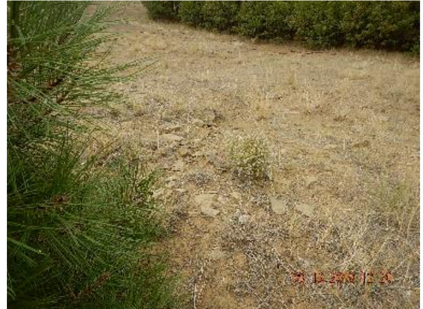
Photo 2: Rills and erosion channeling off fill slope.
