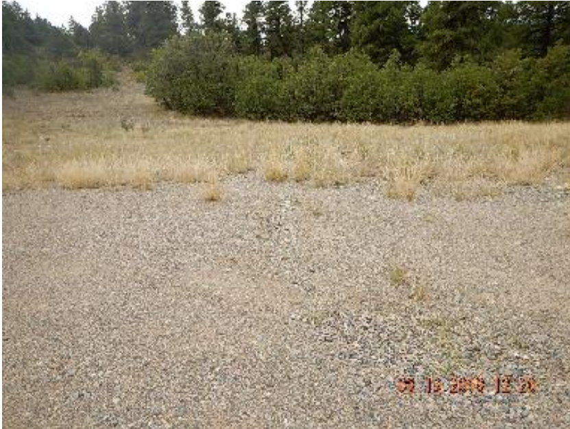
Photo 3: Stormwater channeling in graveled surface.
