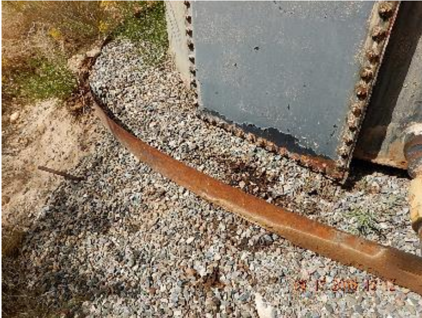
Photo 5: Impacted soil and gravel at production tank man entry hatch.
