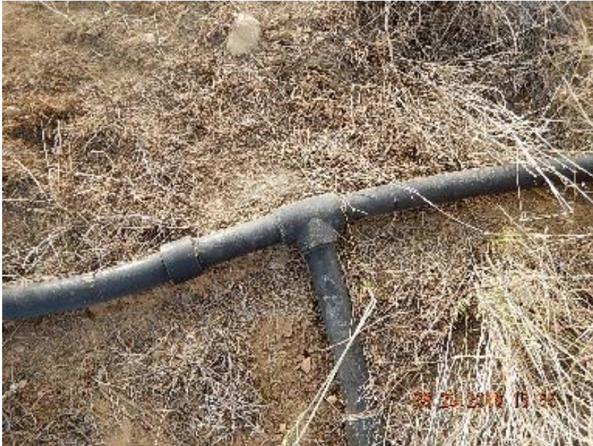
Photo 7: Gathering system black poly line with T that has a split in it.
