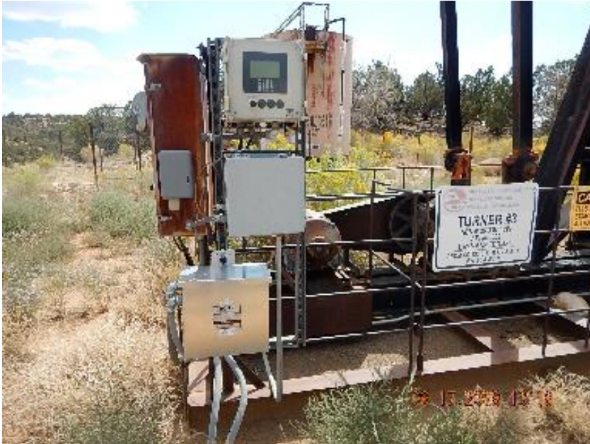
Photo 11: Electrical control equipment at pump jack.
