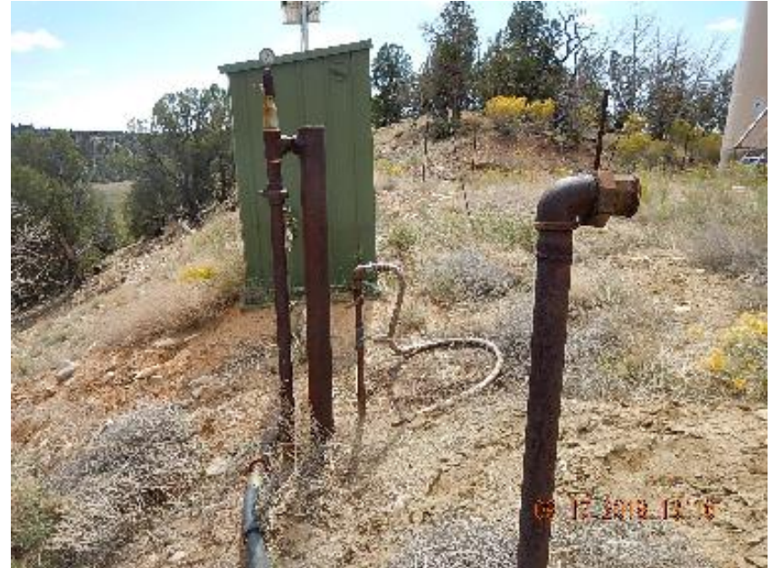
Photo 4: Open ended 3" riser, 1" riser, horseshoe riser, and black poly line at gas meter shed.
