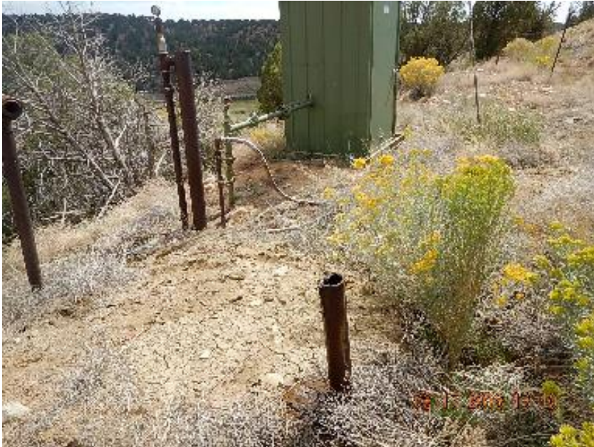
Photo 3: Open ended 3" riser with impacted soil at gas meter shed area.
