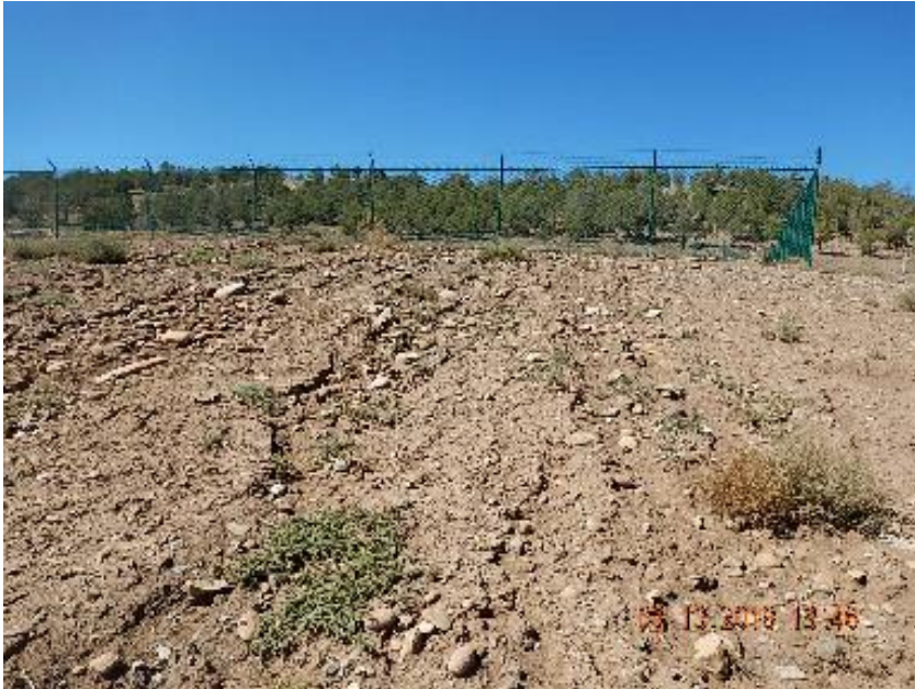
Photo 9: Rilling and erosion on S fill slope.
