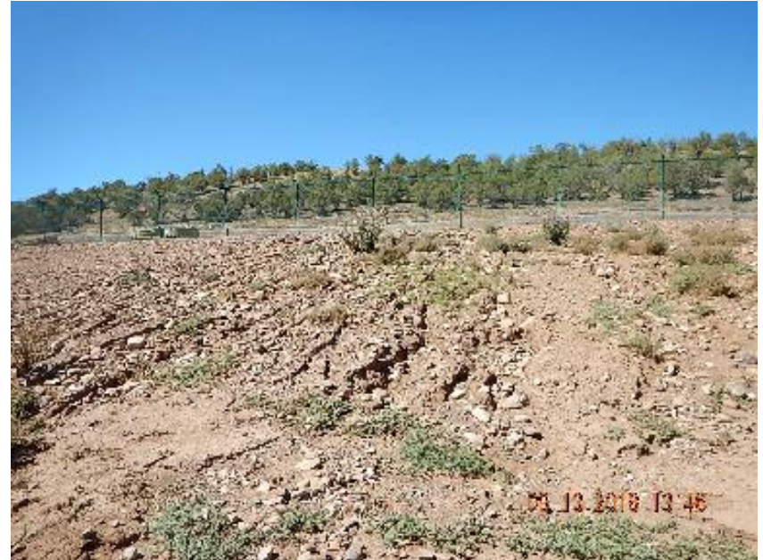
Photo 10: Rilling and erosion on S fill slope.
