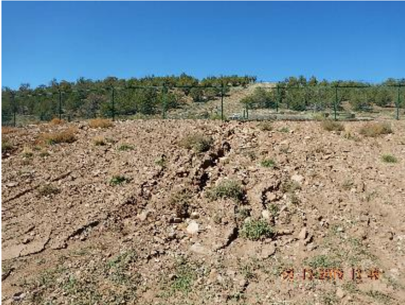
Photo 11: Erosion channel on S fill slope.
