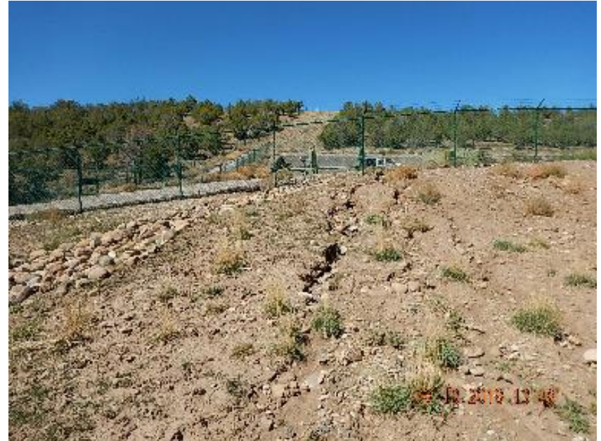
Photo 12: Erosion channel on S fill slope.
