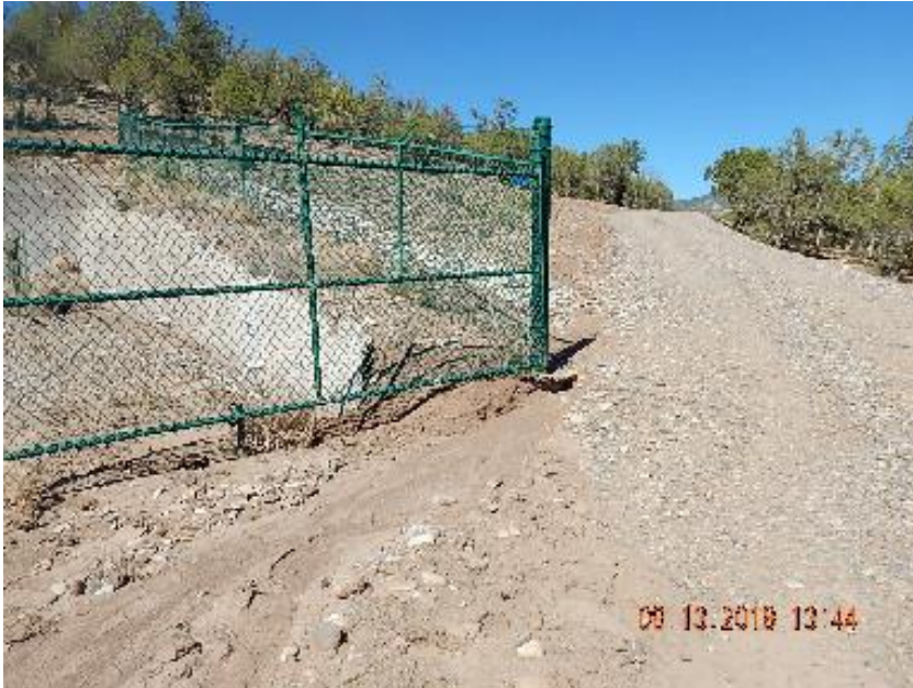
Photo 7: Sediment flow onto location from NE corner cobble run and erosion channel outside cobble.
